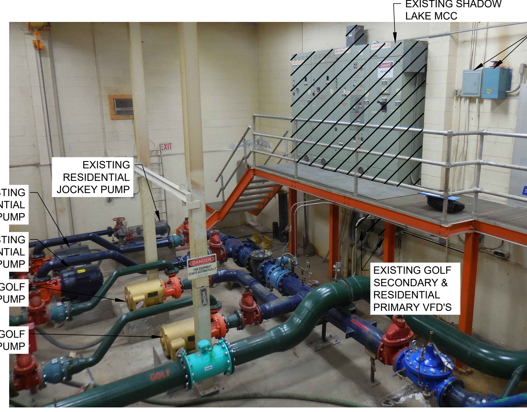
SHADOW LAKE PUMP STATION DEMOLITION DETAIL
