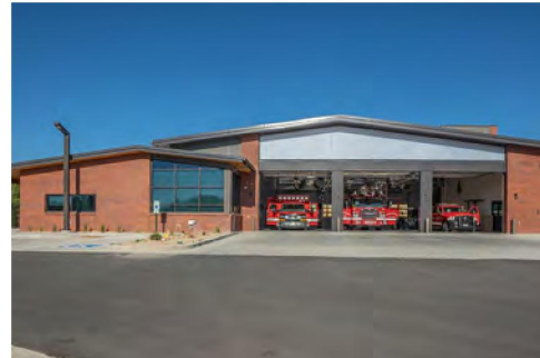
City of Grand Junction Fire Station No. 6 Grand Junction, CO
