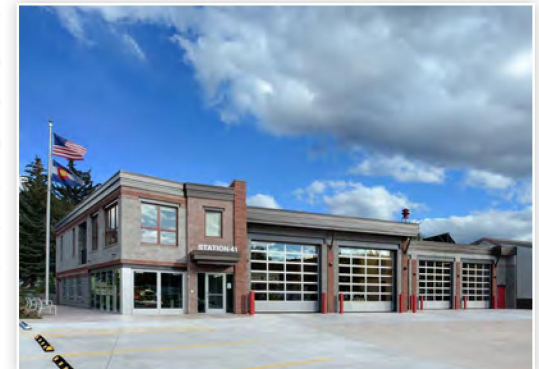
Basalt Fire Station No. 41
