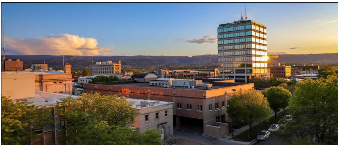
Alpine Bank Tower
