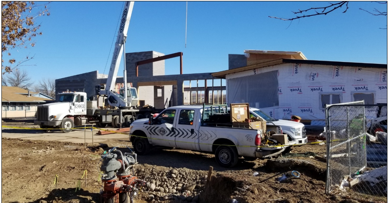
Fire Station 3 Under Construction
