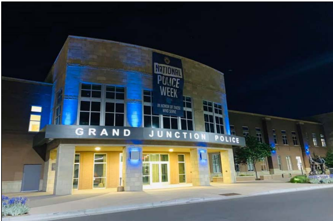
Grand Junction Police Department and 9-1-1 Communications Center Building
