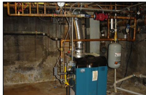
Facilities Projects done in 2019
