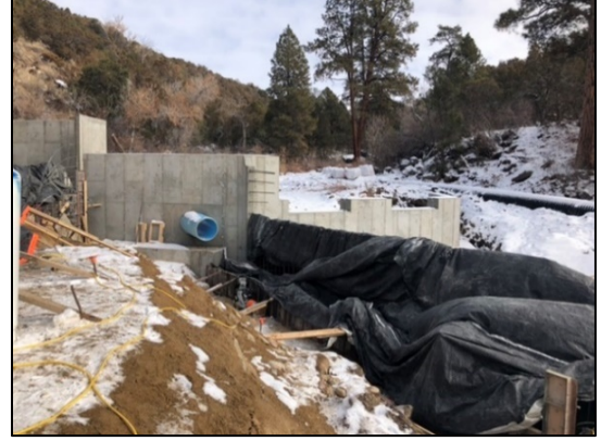
New Kannah Creek Intake Structure
