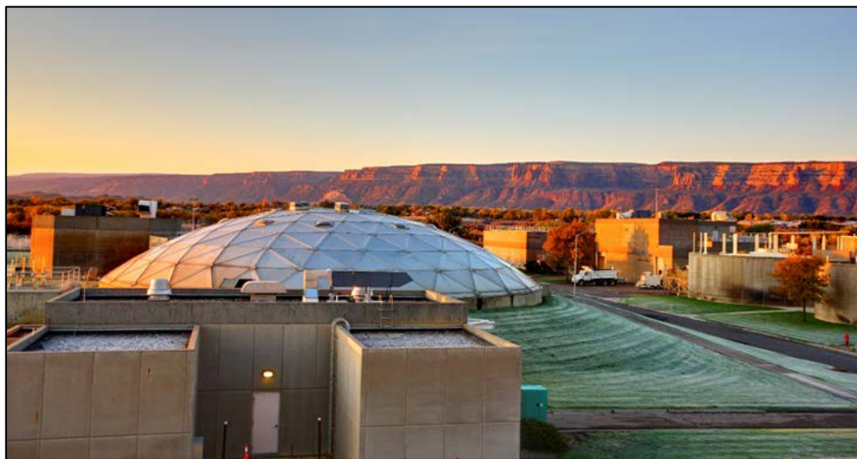
City of Grand Junction Wastewater Treatment Facility
