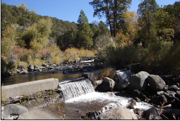
Old Kannah Creek Intake Structure
