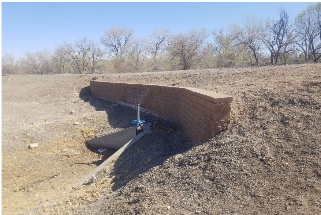
Figure 12: Retaining Wall at Stormwater Detention Pond C
