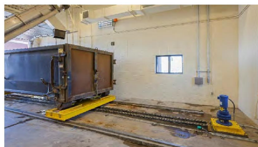
Figure C-6. Load leveling Dumpster Veyor at the Stonegate WWTP
