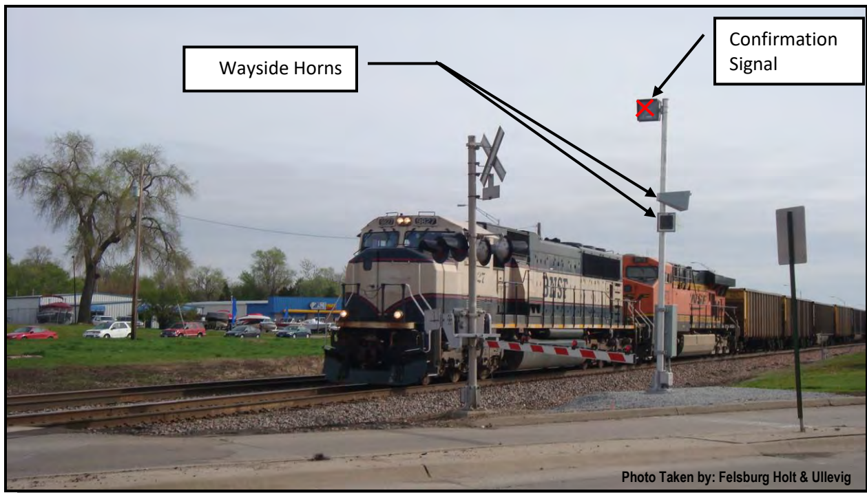
Figure 3. Highway-Rail Crossing Equipped with Wayside Horns
