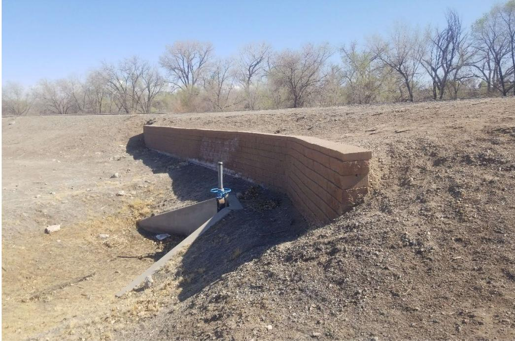
**Figure 12: Retaining Wall at Stormwater Detention Pond C**
