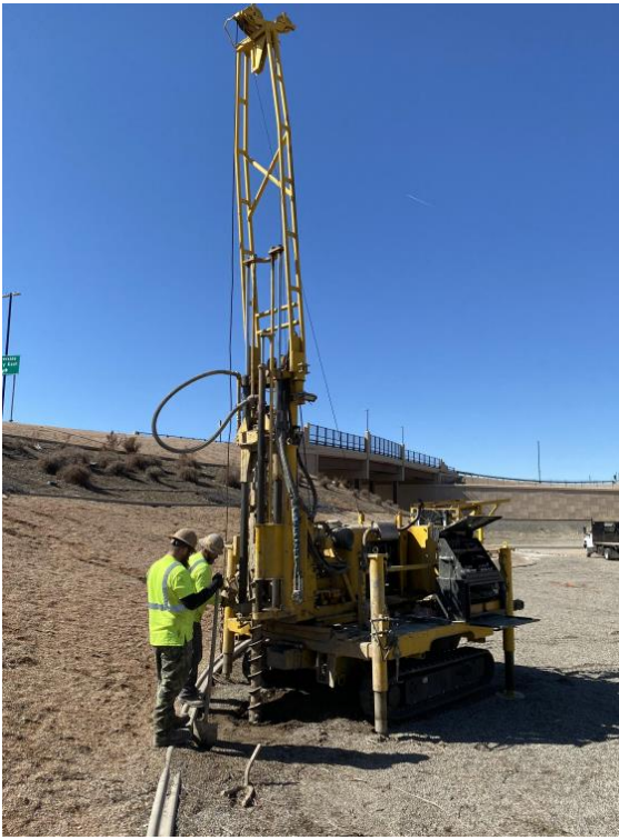
Borehole B-6 Site Two 12" Duct Toe of Embankment
