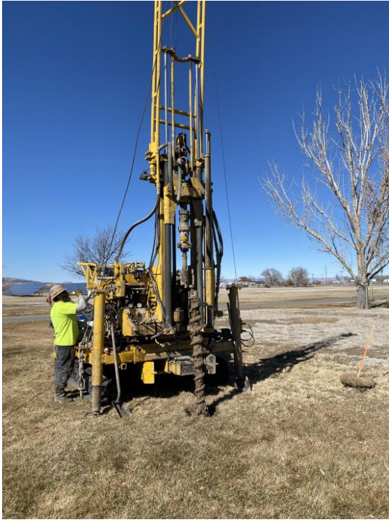
Borehole B-2 Site One Bio Filter Pad Number 2 NW
