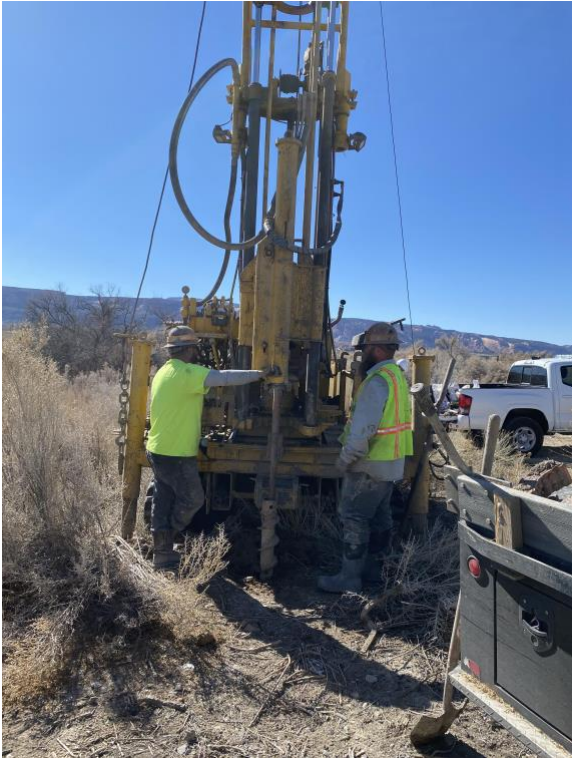
Borehole B-3 & B-4 General Location of Site One Aerial Pipe Crossing
