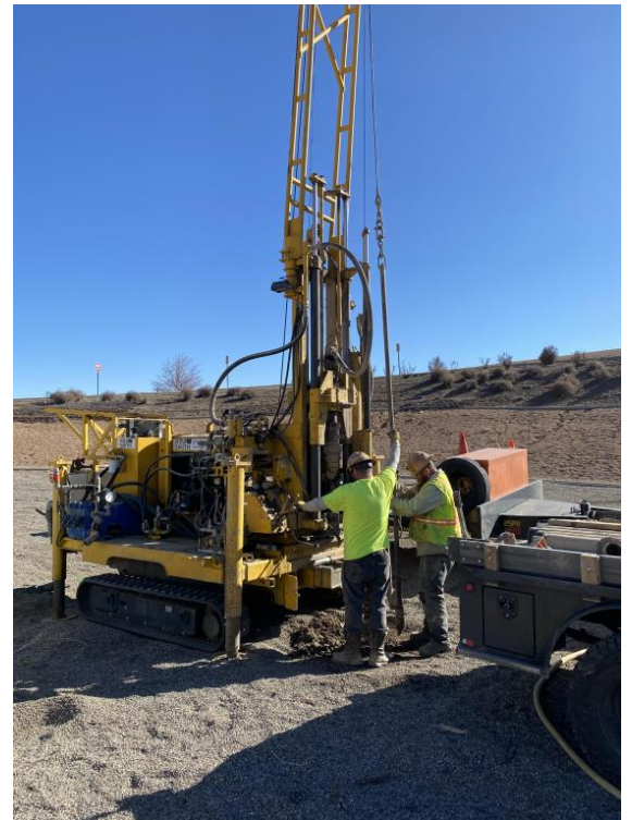
Borehole B-5 Site Two Bio Filter Pad Number 2 (Dos Rios)
