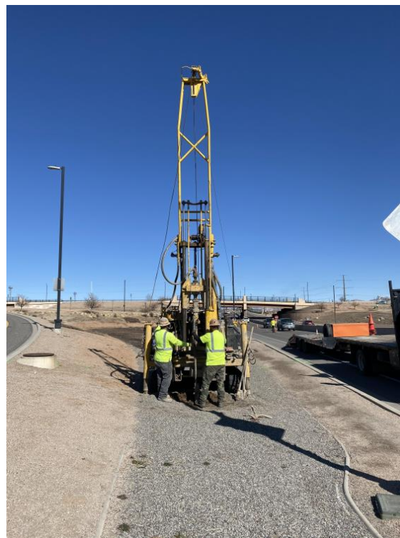
Borehole B-7 Site Two 12" Duct near Manhole tie in
