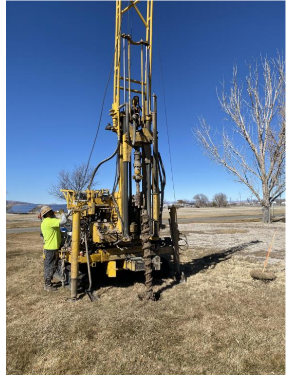
Borehole B-2 Site One Bio Filter Pad Number 2 NW
