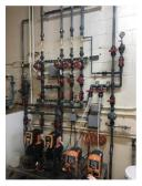
JVA designed improvements to the District's 3 MGD South Water Treatment Plant (SWTP) which included replacing the onsite sodium hypochlorite generation system, relining an existing FRP tank to store 5,000 gallons of sodium hypochlorite,
