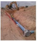
JVA has been providing numerous water projects for the District. This recent pipeline project included approximately 11,000 linear feet of water transmission main from the Water Treatment Plant to South
