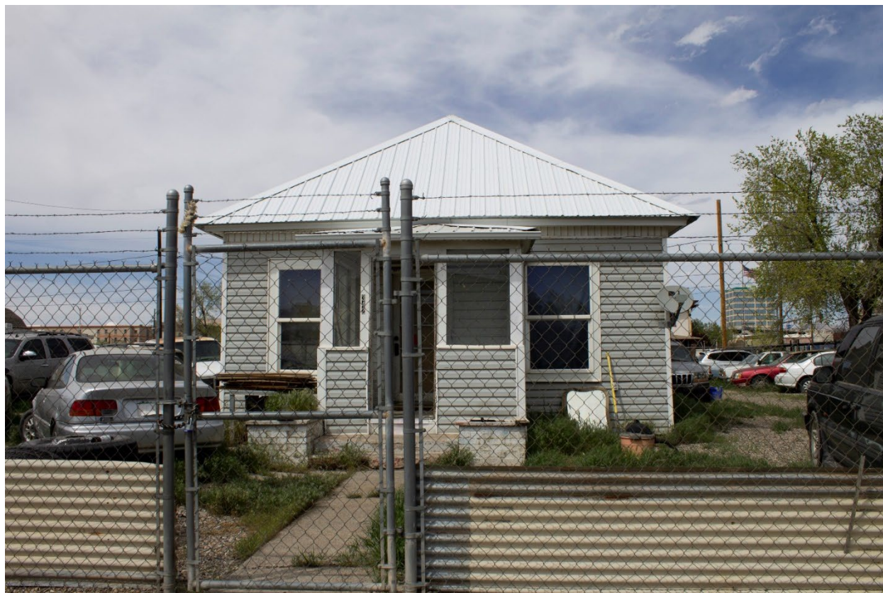
Figure 63. 342 Pitkin Avenue (5ME.8640). View to the north. April 2022
