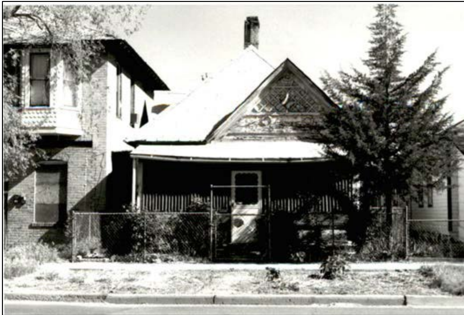
Figure 58. 242 Pitkin Avenue (5ME.8646). View to the north. This image is found in the property's 1996 site record prepared by the Museum of Western Colorado. Note the chimney and the ornamentation on the front cross-gable.
