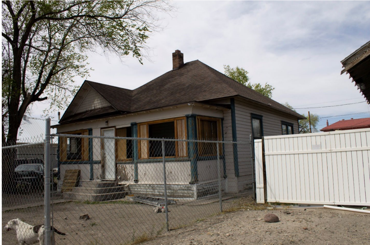
Figure 65. 352 Pitkin Avenue (5ME.8641). View to the northwest. April 2022
