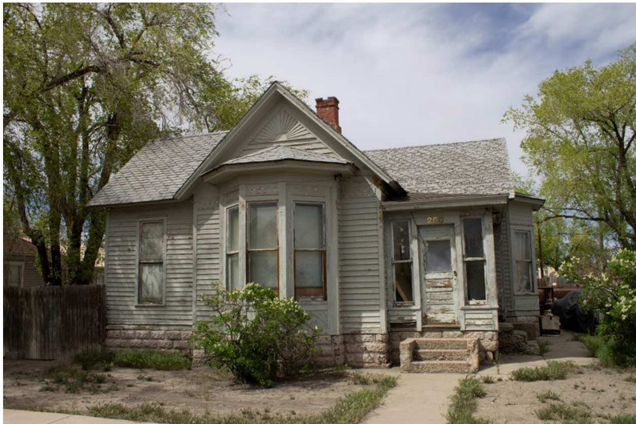
Figure 40. 260 Pitkin Avenue (5ME.7766). View to the north. April 2022
