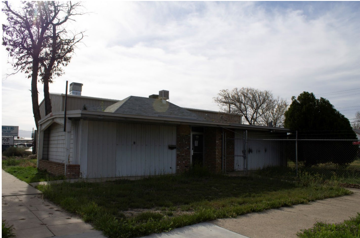
Figure 66. 309 Pitkin Avenue (5ME.23878). View to the southeast. April 2022
