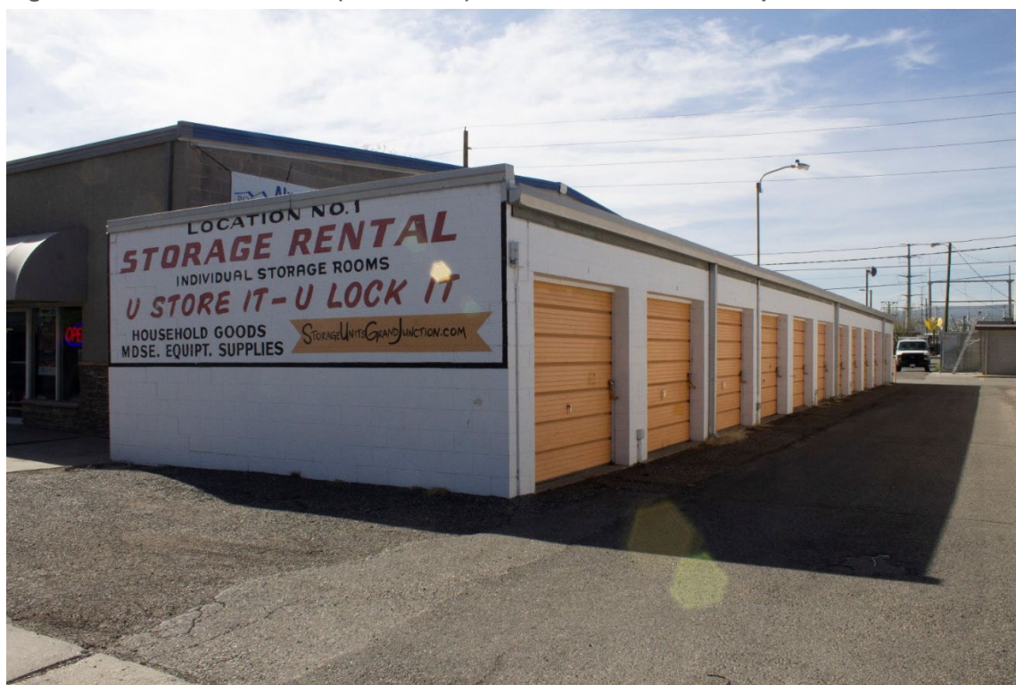
Figure 71. 523 Pitkin Avenue (5ME.23880). View to the southeast. April 2022
