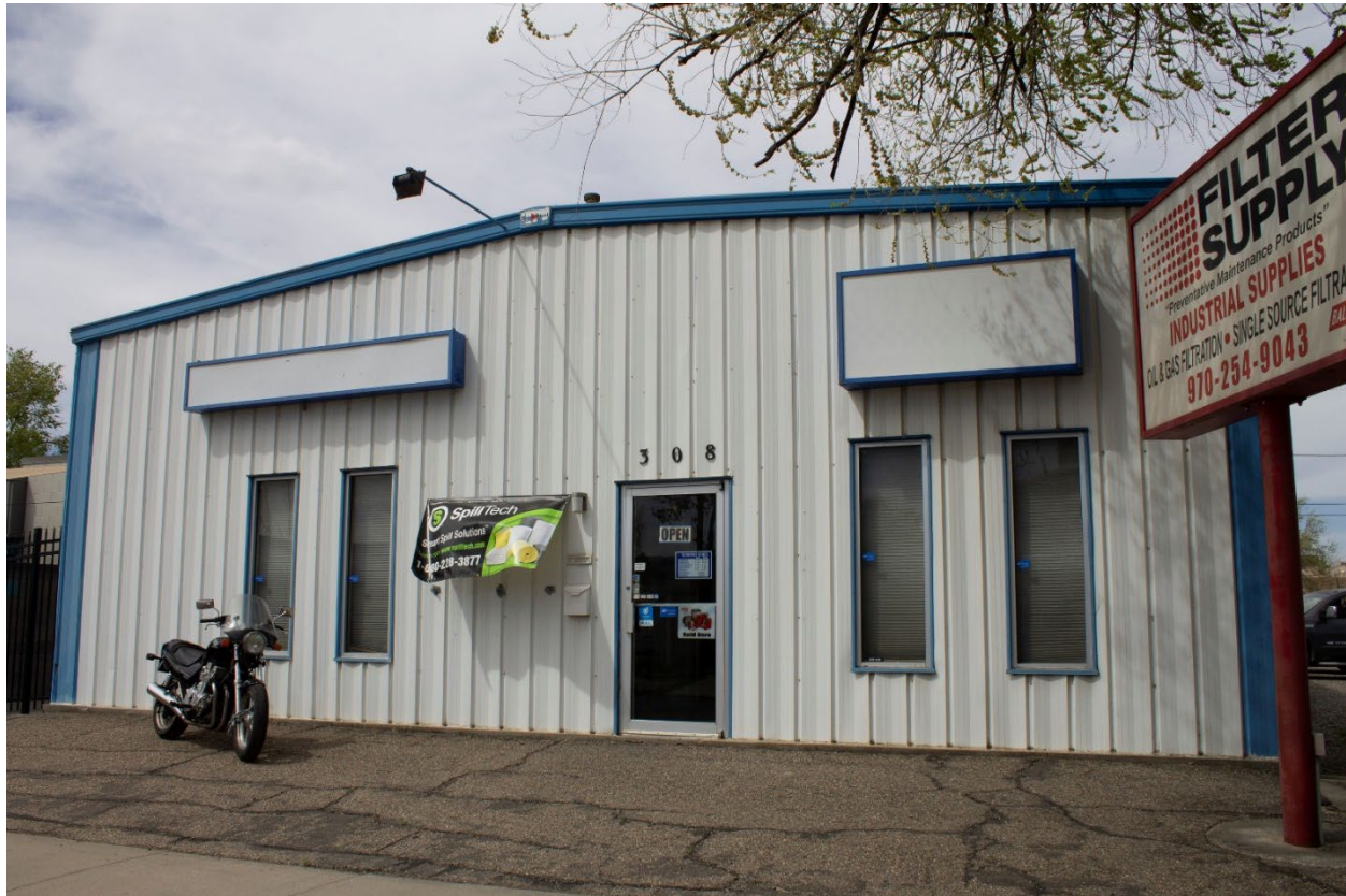
Figure 62. 308 Pitkin Avenue (5ME.23875). View to the north. April 2022
