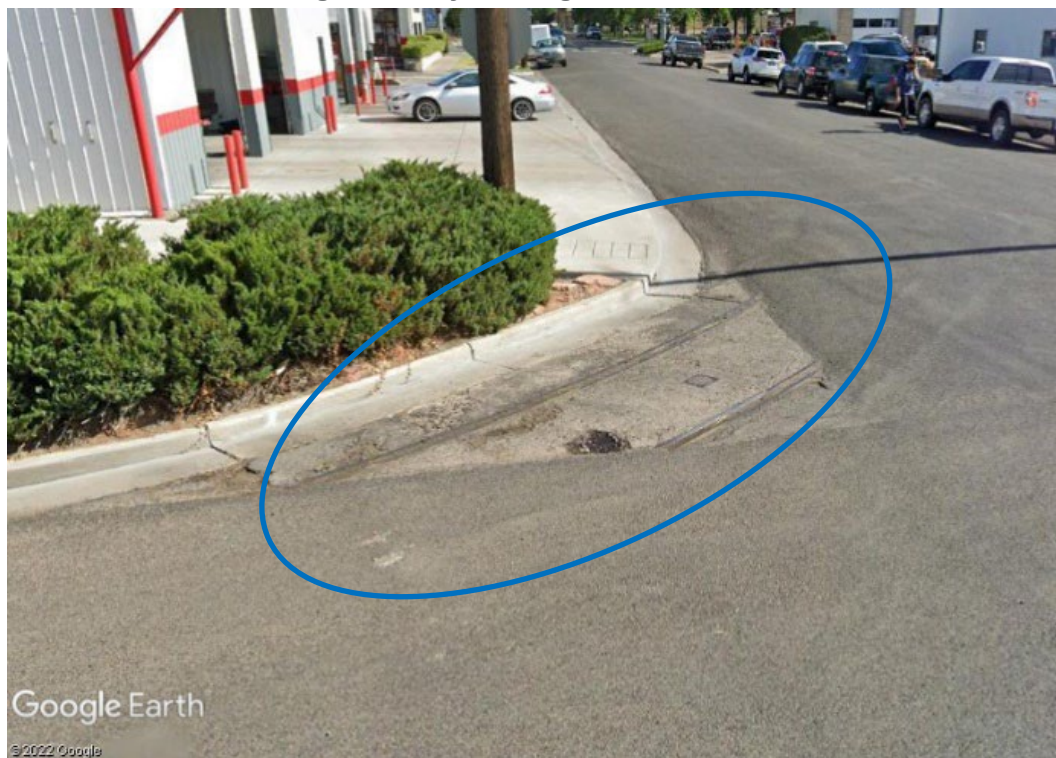
Figure 48. 5ME.24074.1. Exposed streetcar tracks at the northwest corner of 4th Street and South Avenue. View north. Image courtesy of Google Earth.
