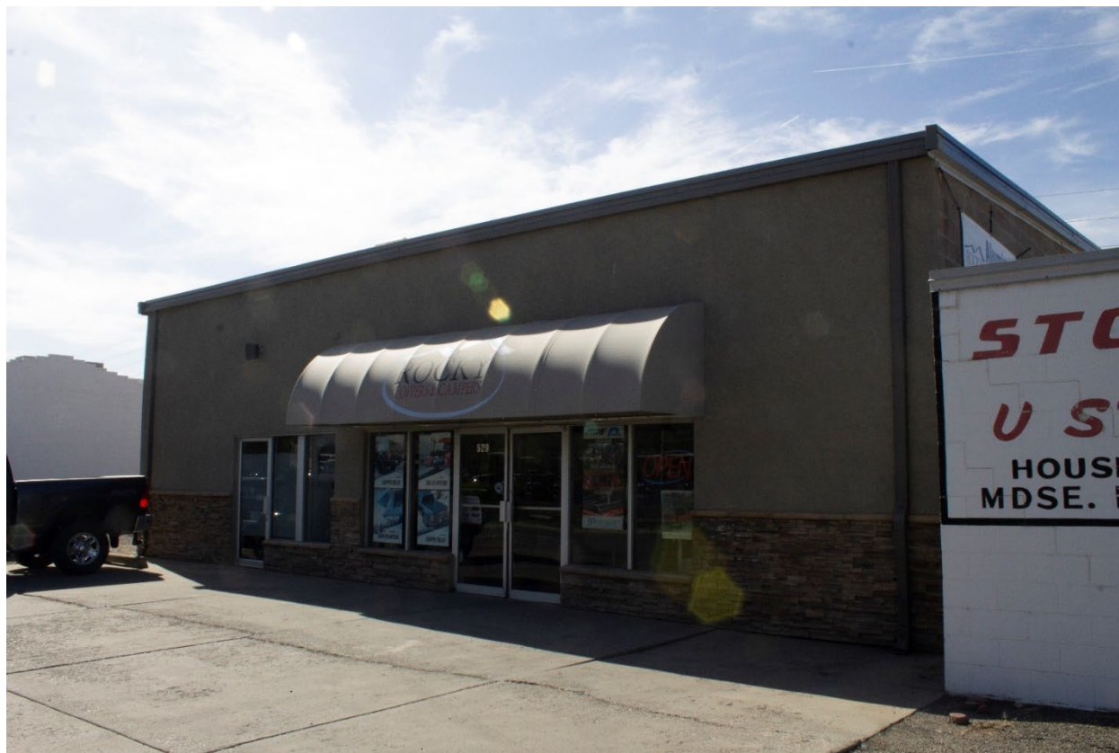
Figure 73. 529 Pitkin Avenue (5ME.23881). View to the southeast. April 2022
