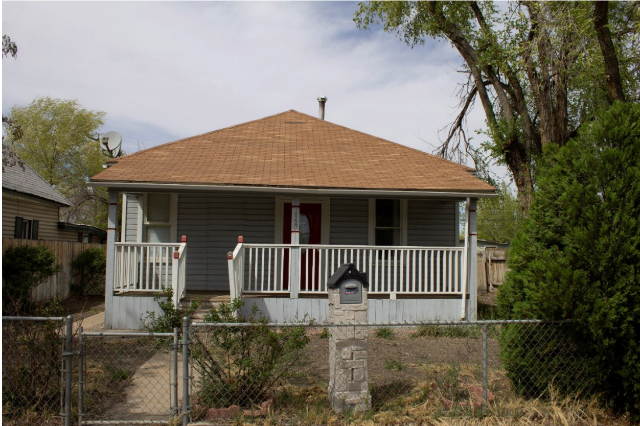
Figure 59. 244 Pitkin Avenue (5ME.8647). View to the north. April 2022
