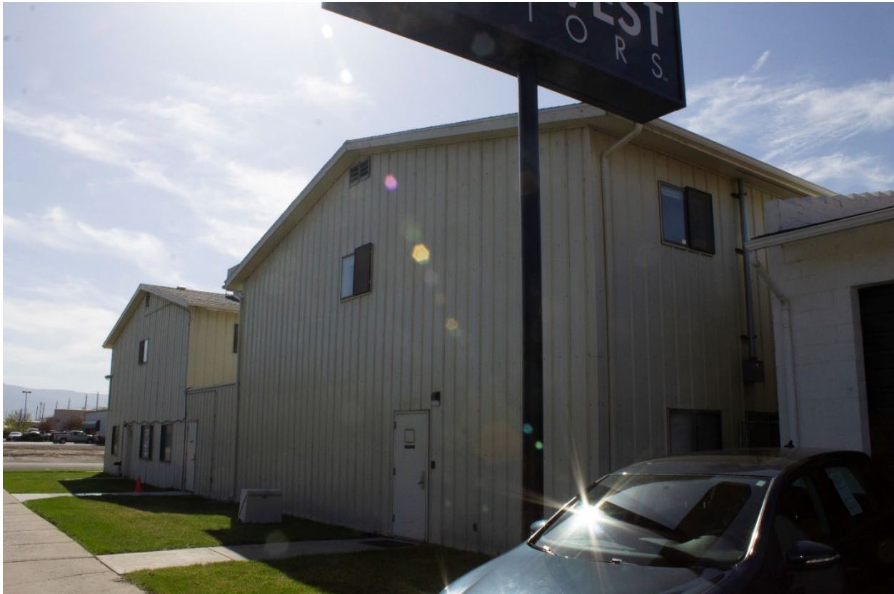
Figure 74. 549 Pitkin Avenue (5ME.23882). View to the southeast. April 2022
