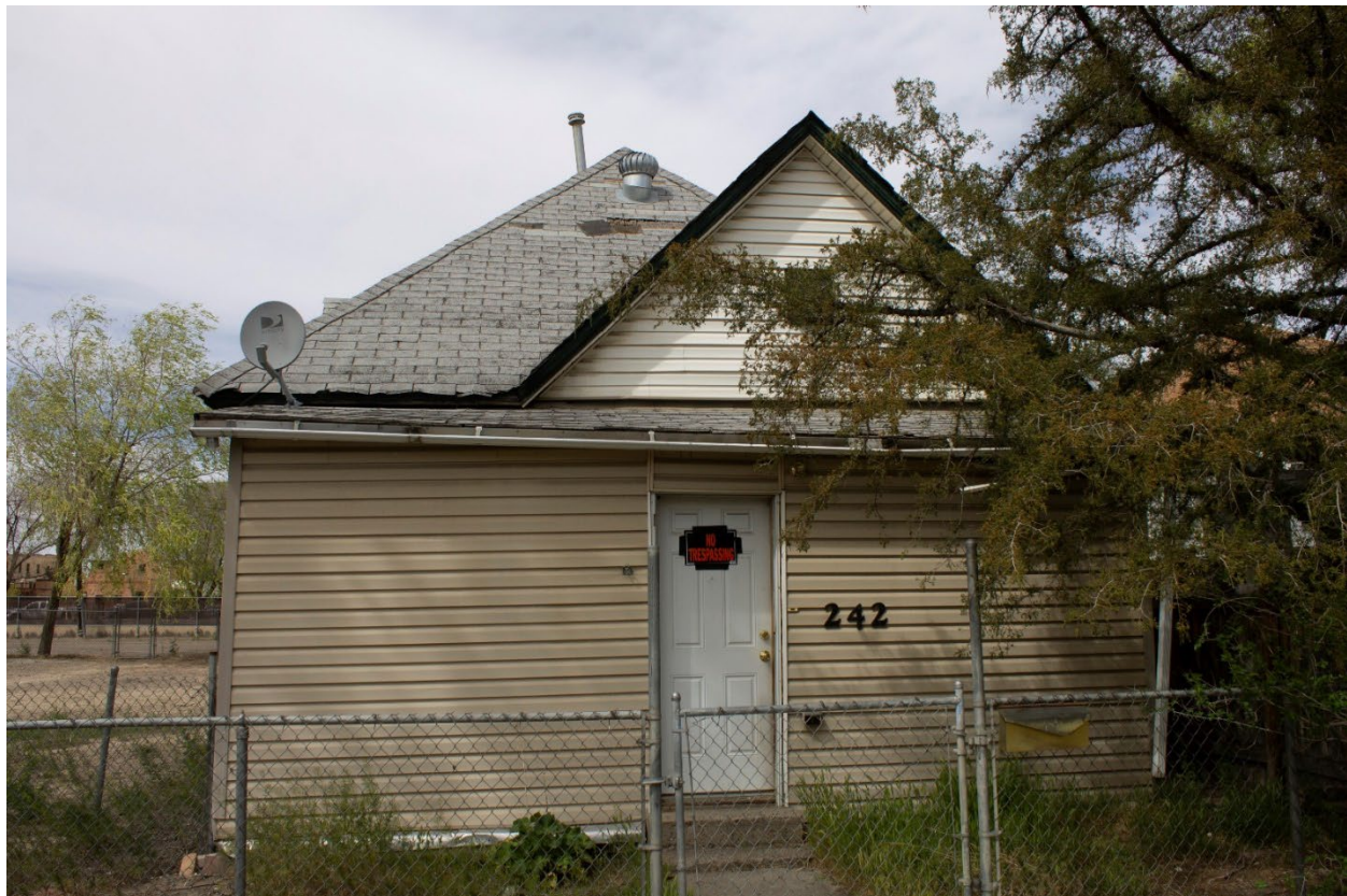
Figure 57. 242 Pitkin Avenue (5ME.8646). View to the north. April 2022
