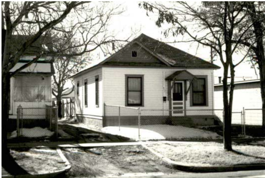
Figure 68. 319 Pitkin Avenue (5ME.7768). View to the southwest. This image is found in the property's 1996 site record prepared by the Museum of Western Colorado. Note the windows and front entry.
