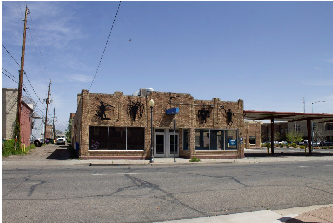
Figure 14. Bus terminal for the Rio Grande Motor Way. April 2022.
