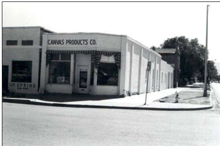
Figure 55. 338 South 2nd Street (5ME.4146). View to the east. This image is found in the property's 1982 site record prepared by Robin Krawitz. Note the original commercial storefront with a central recessed single-door entrance flanked by large display windows.
