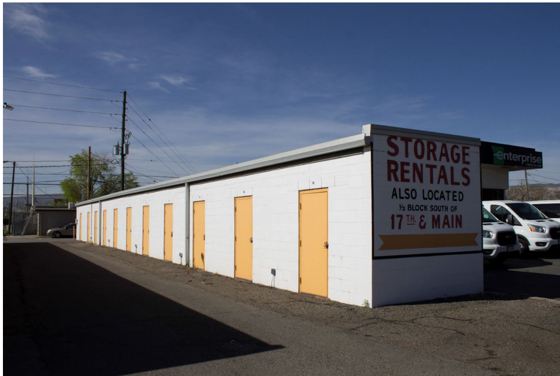
Figure 72. 523 Pitkin Avenue (5ME.23880). View to the southwest. April 2022
