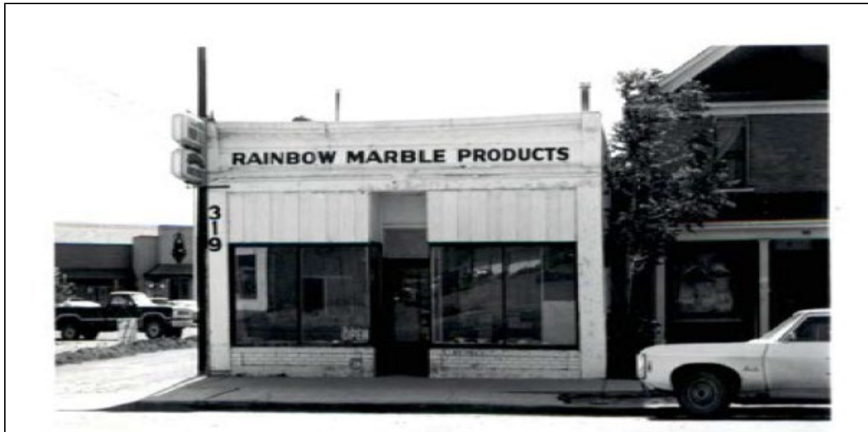
Figure 51. 319 South 2nd Street (5ME.4145). East elevation. View to the west. This image is found in the property's 1982 site record prepared by Robin Krawitz. Note the adjacent building to the north and the modern display glass.
