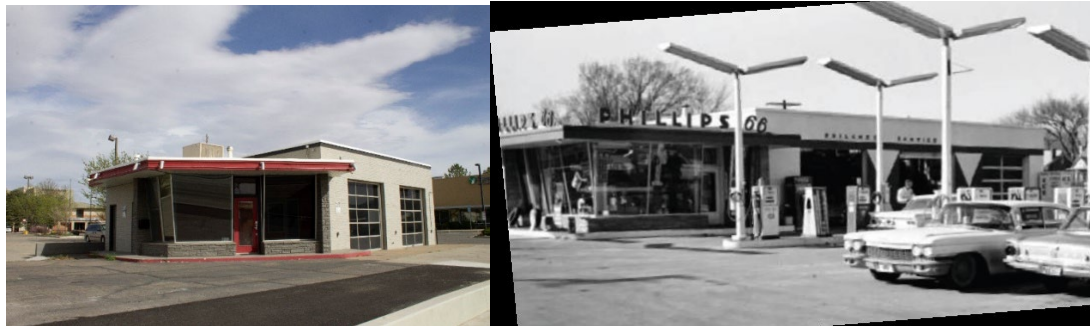
Figure 17. Left: Formerly Don & Mel's 66 Service Station built in 1956 according to Phillips 66 standard designs of the time. This building would have originally featured prominent signage and gas pumps. Photo taken in April 2022. Right: An example of a similar standardized Phillips 66 station located in Tulsa, Oklahoma (photograph found in Jones 2016, 7-12).
