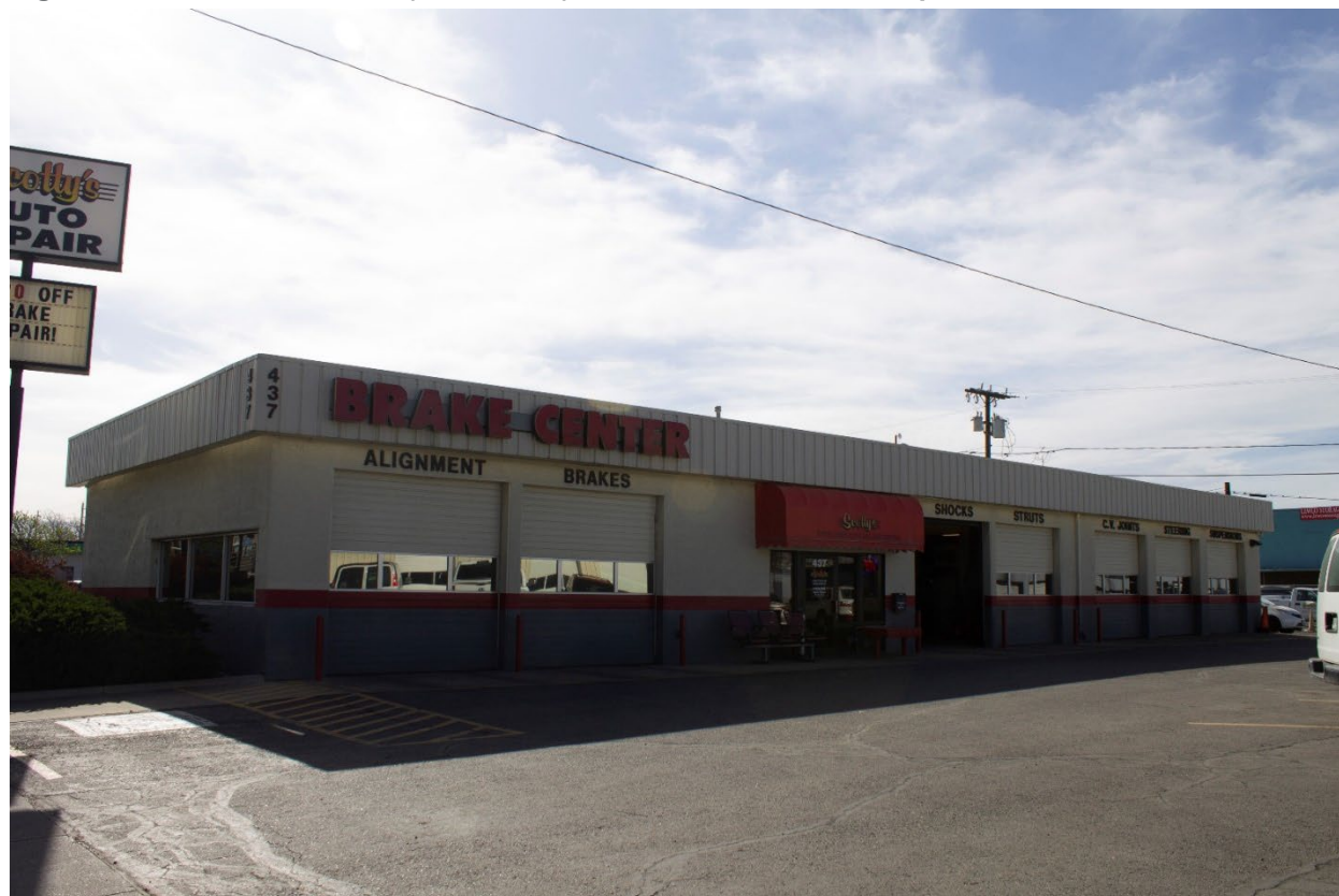
Figure 70. 437 Pitkin Avenue (5ME.23884). View to the southeast. April 2022
