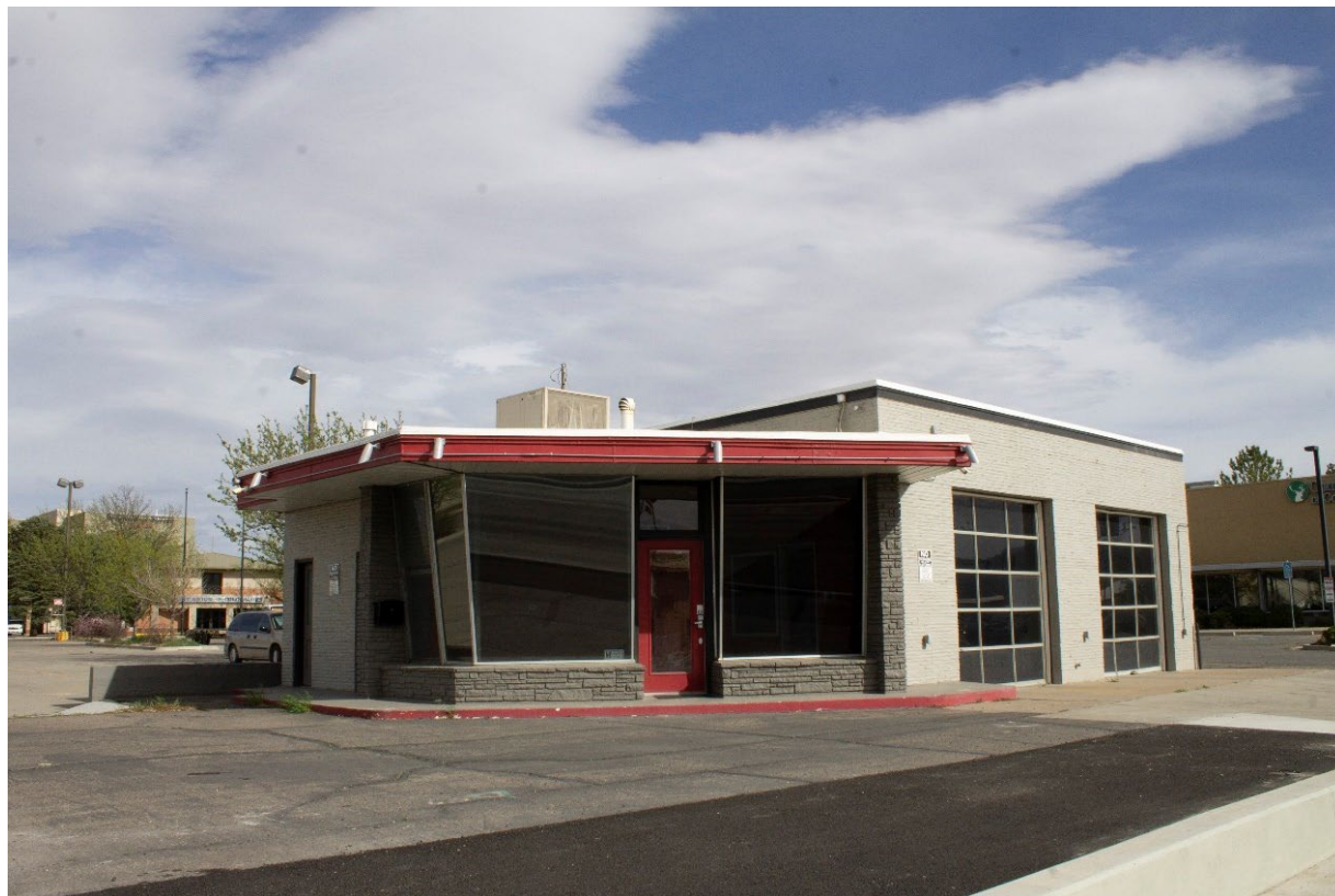
Figure 21. 124 North 1st Street (5ME.15689). Front elevation. View to southeast. April 2022
