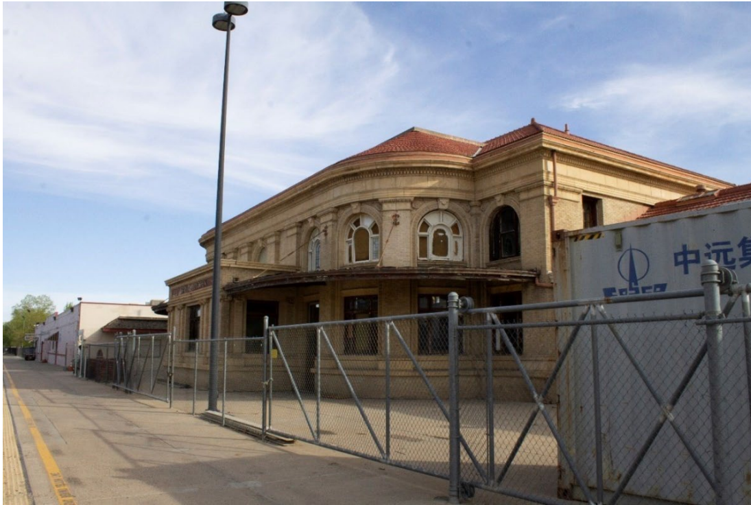
Figure 34. 119 Pitkin Avenue (5ME.4163). Track side (southwest) elevation. View to the north. April 2022
