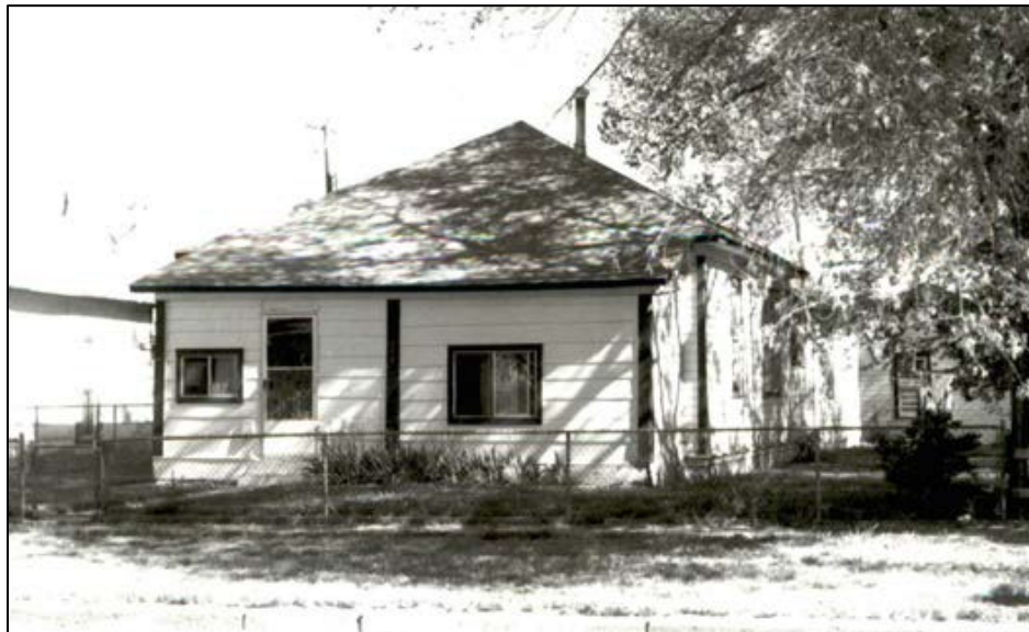
Figure 60. 244 Pitkin Avenue (5ME.8647). View to the northwest. This image is found in the property's 1996 site record prepared by the Museum of Western Colorado. Note the enclosed front porch.
