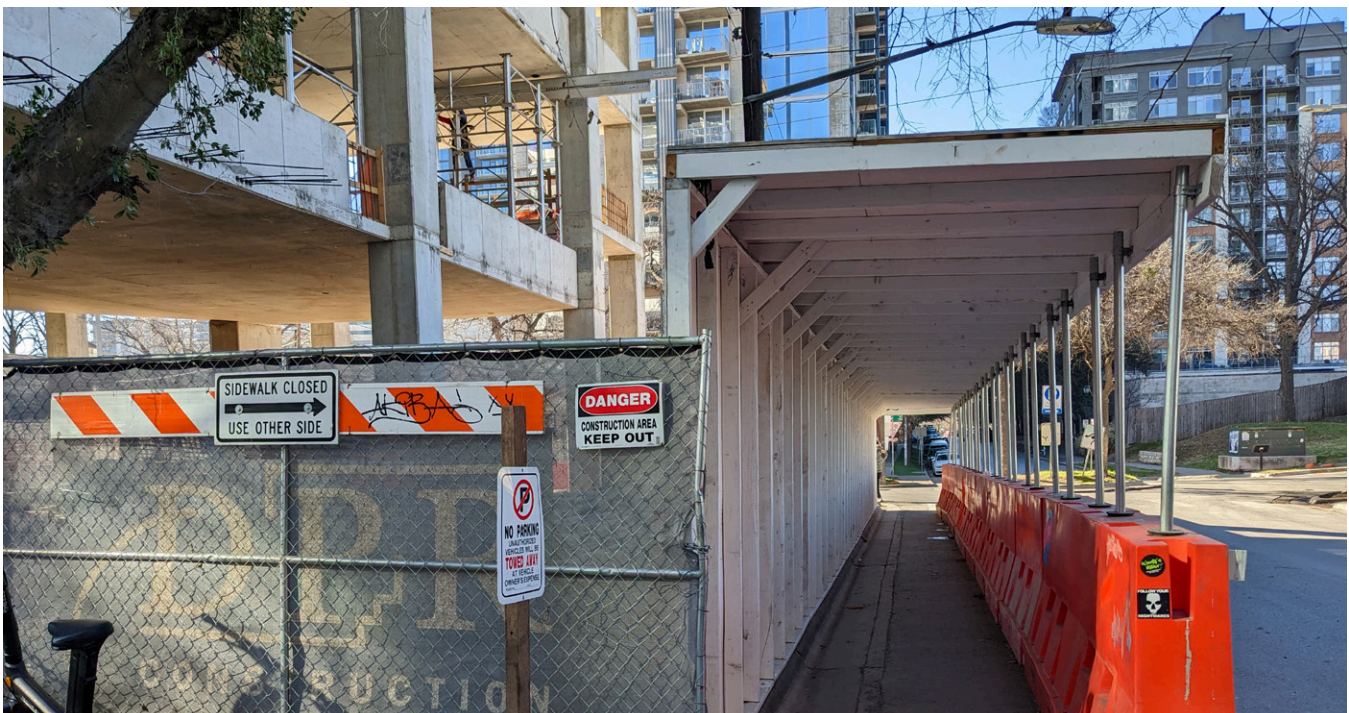
FIGURE 43: EXAMPLE OF COVERED WALKWAY AT CONSTRUCTION SITE
