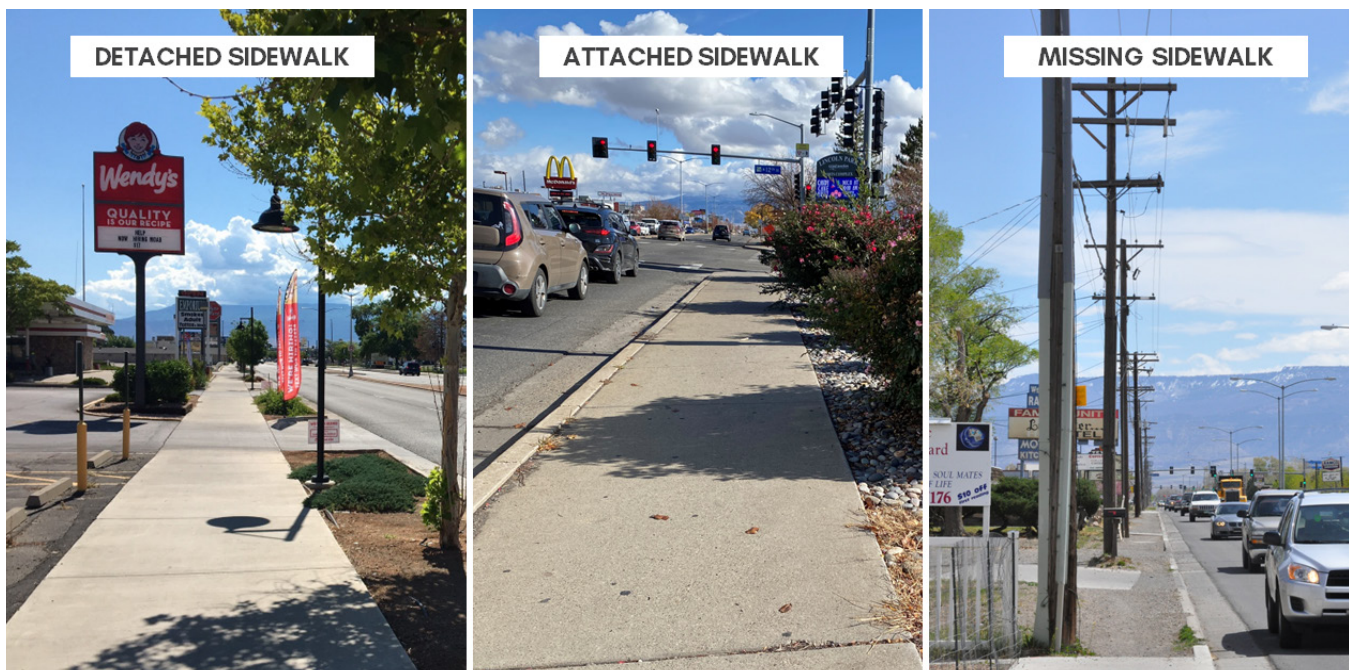
FIGURE 1: EXISTING SIDEWALK TYPES MAPPED IN GRAND JUNCTION
