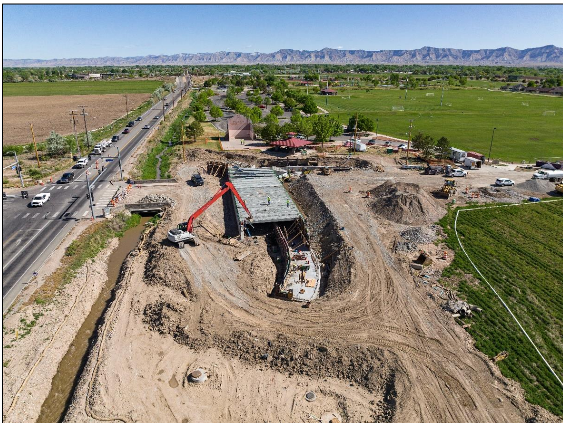
24 Road and G Road Bridge Construction
