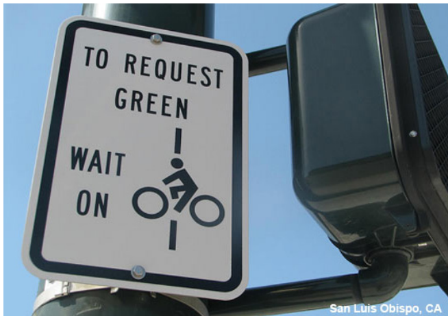
FIGURE 27 BIKE DETECTION AT SIGNAL
