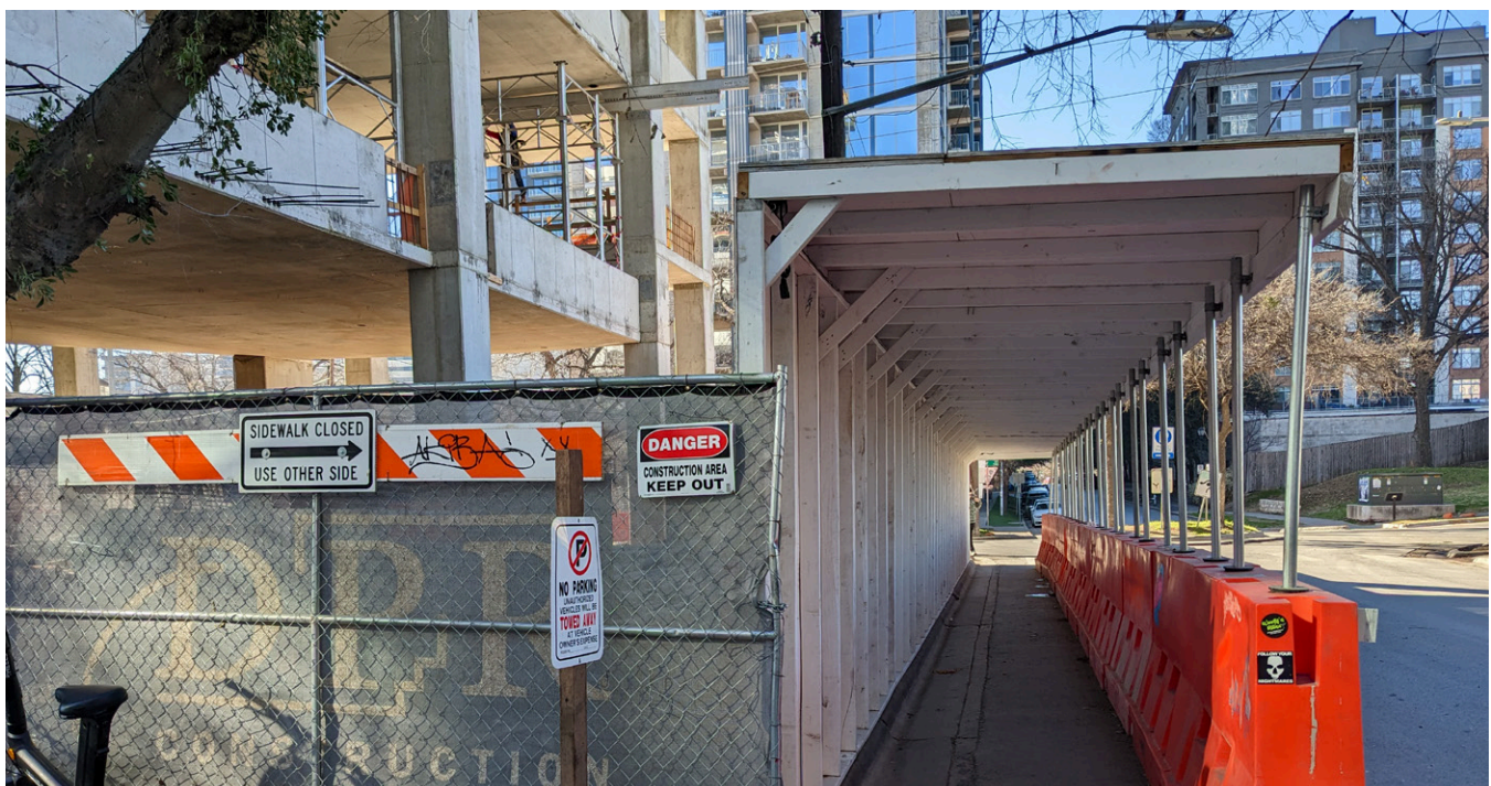
FIGURE 43: EXAMPLE OF COVERED WALKWAY AT CONSTRUCTION SITE
