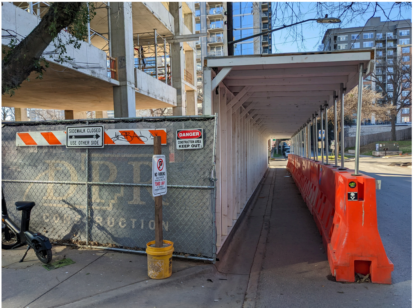
FIGURE 43: EXAMPLE OF COVERED WALKWAY AT CONSTRUCTION SITE
