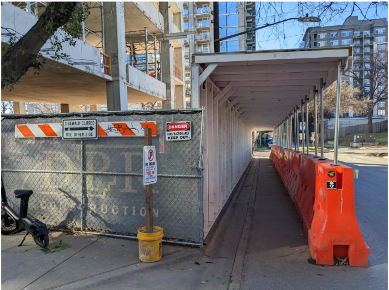
FIGURE 43: EXAMPLE OF COVERED WALKWAY AT CONSTRUCTION SITE
