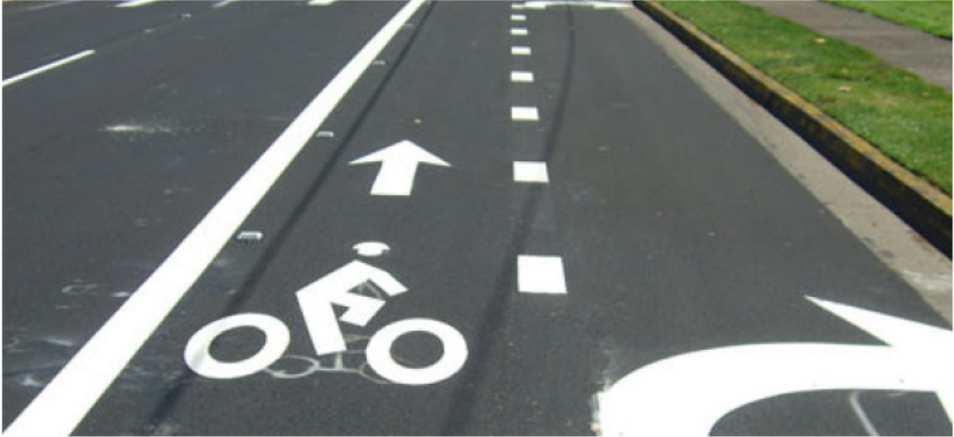
FIGURE 26: COMBINED BIKE LANE/TURN LANE
