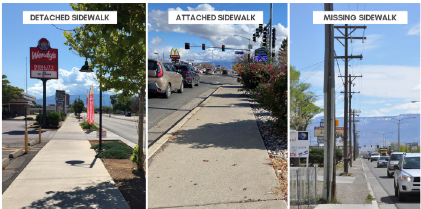
FIGURE 1: EXISTING SIDEWALK TYPES MAPPED IN GRAND JUNCTION
