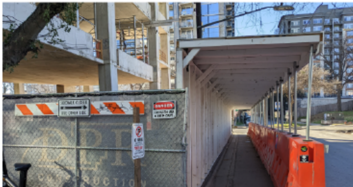
FIGURE 43: EXAMPLE OF COVERED WALKWAY AT CONSTRUCTION SITE
