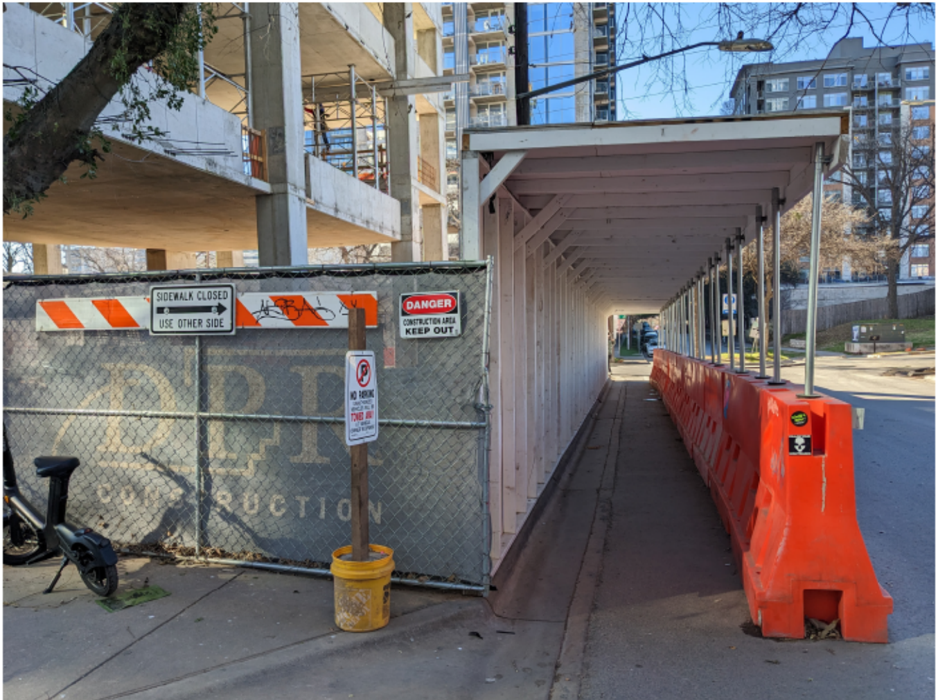
FIGURE 43: EXAMPLE OF COVERED WALKWAY AT CONSTRUCTION SITE
