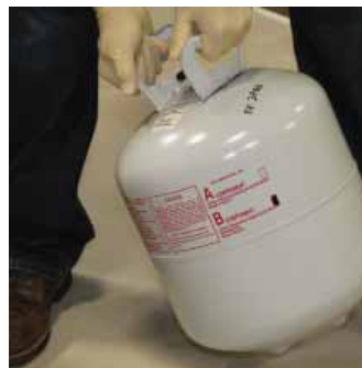
Shaking of A-side and B-side tanks
