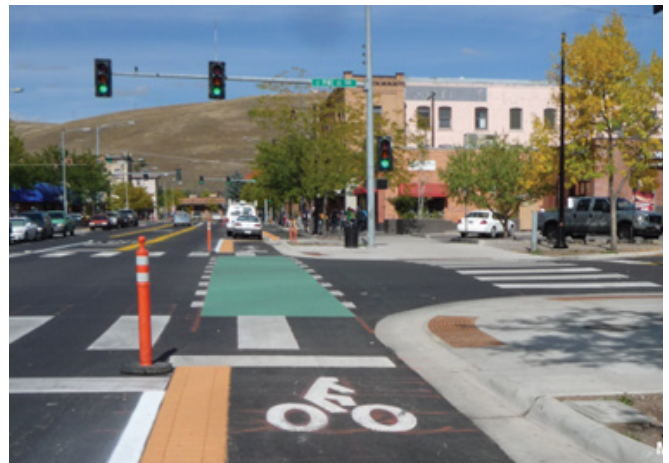
FIGURE 28: RECESSED STOP BAR
