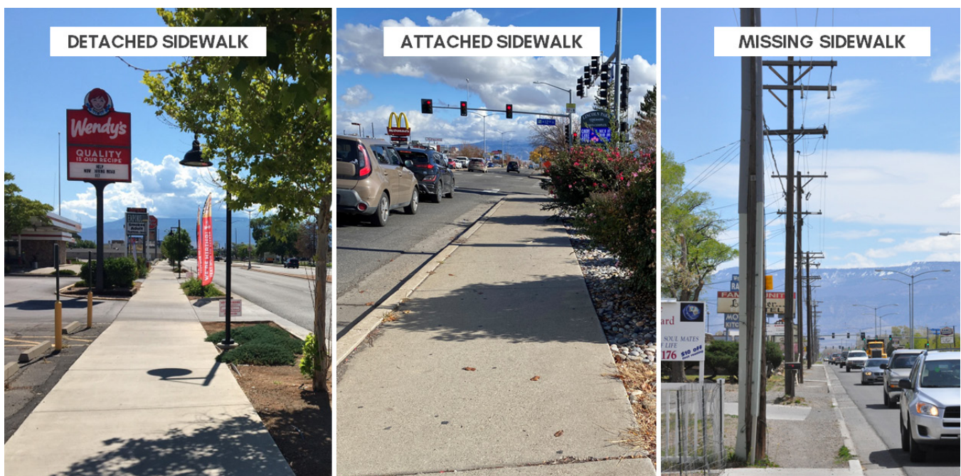
FIGURE 1: EXISTING SIDEWALK TYPES MAPPED IN GRAND JUNCTION
