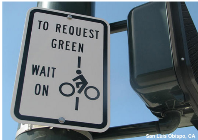
FIGURE 27: BIKE DETECTION AT SIGNAL
