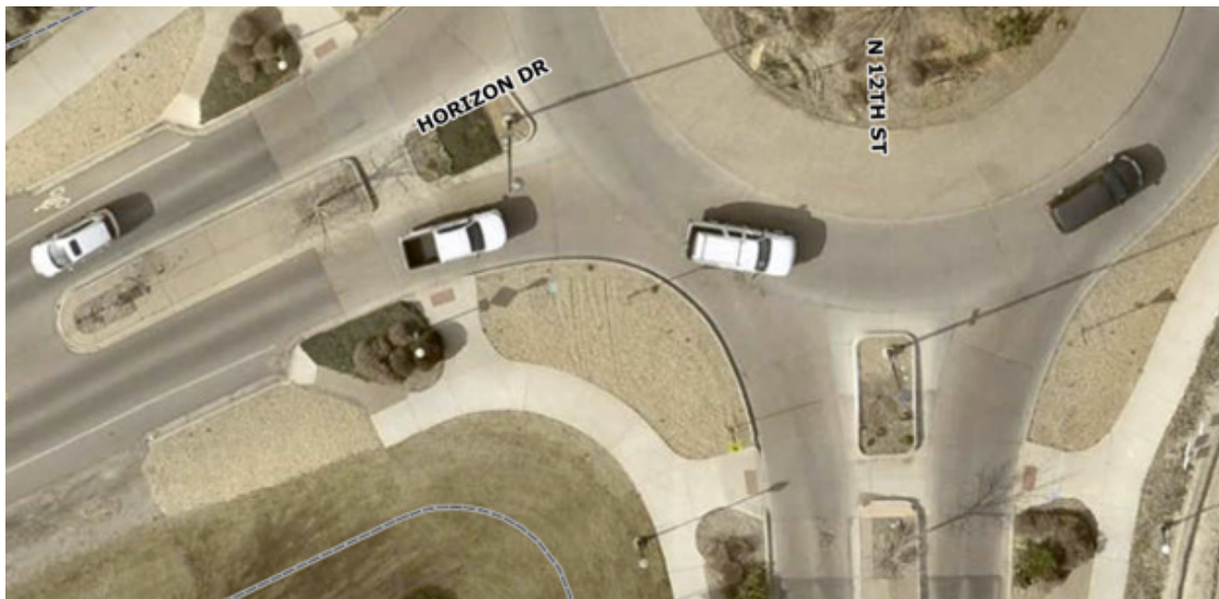
FIGURE 24: BIKE LANE RAMPS AT 12TH STREET AND HORIZON DRIVE ROUNDABOUT
