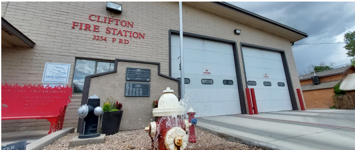
Figure 9 The CFPD station would need a few updates for uniformity and serviceability under a cooperative service agreement.
