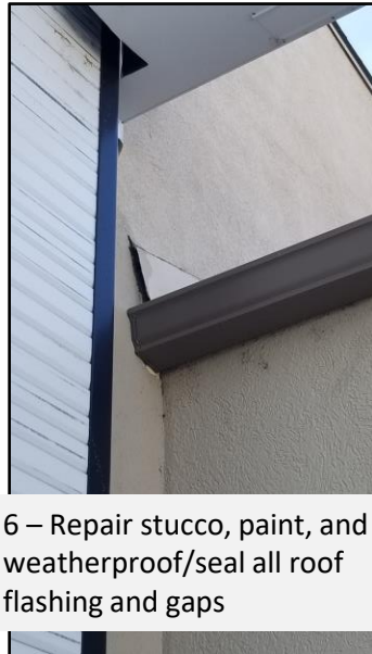
2 – Stucco repair and paint
