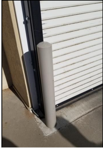
1 – Paint ALL Bollards Yellow (7 total)
