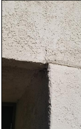
3 – Stucco repair and paint
