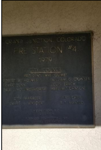
2 – Remove plaque, patch stucco and paint
