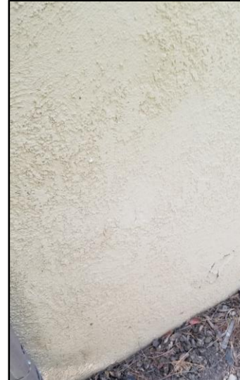
4 – Stucco repair and paint
