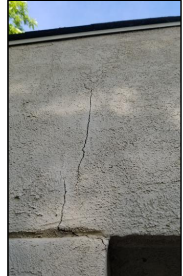
5 – Stucco repair and paint
