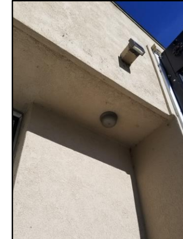
3 – Remove mounted bell, patch stucco and paint
