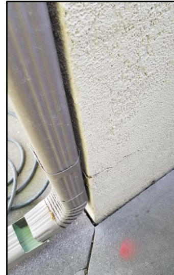
9 – Stucco repair and paint
