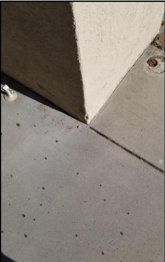
6 – Stucco repair and paint
