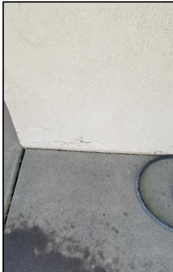
7 – Stucco repair and paint
