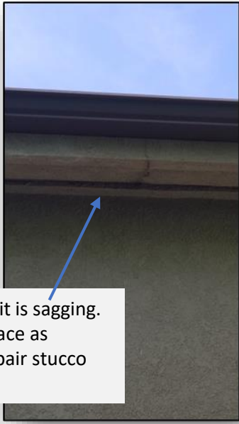
3 – Stucco repair and paint
