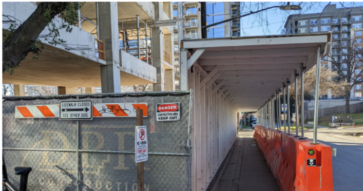
FIGURE 43: EXAMPLE OF COVERED WALKWAY AT CONSTRUCTION SITE
