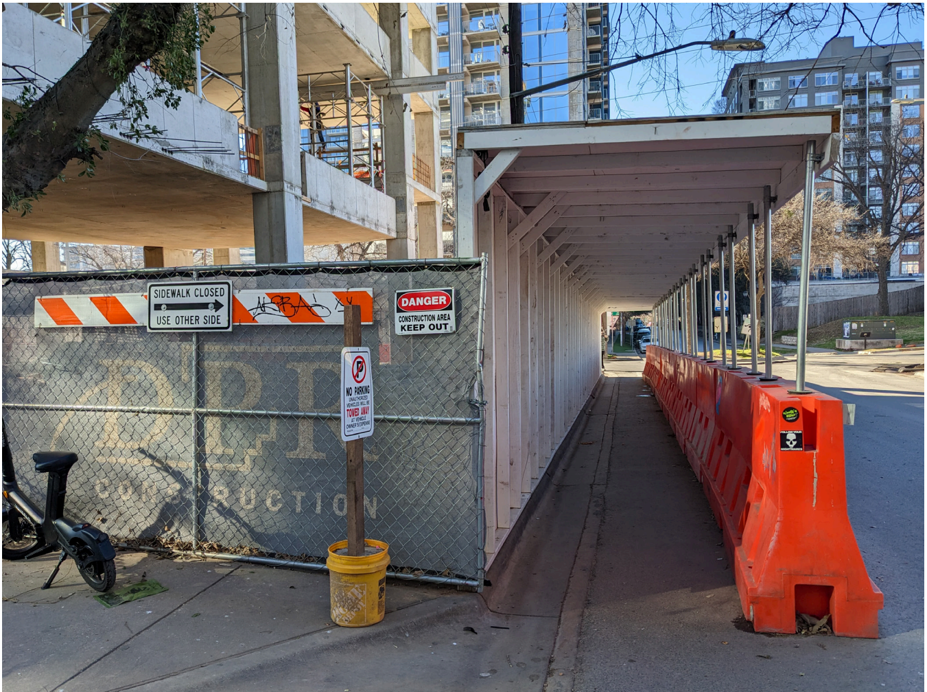
FIGURE 43: EXAMPLE OF COVERED WALKWAY AT CONSTRUCTION SITE
