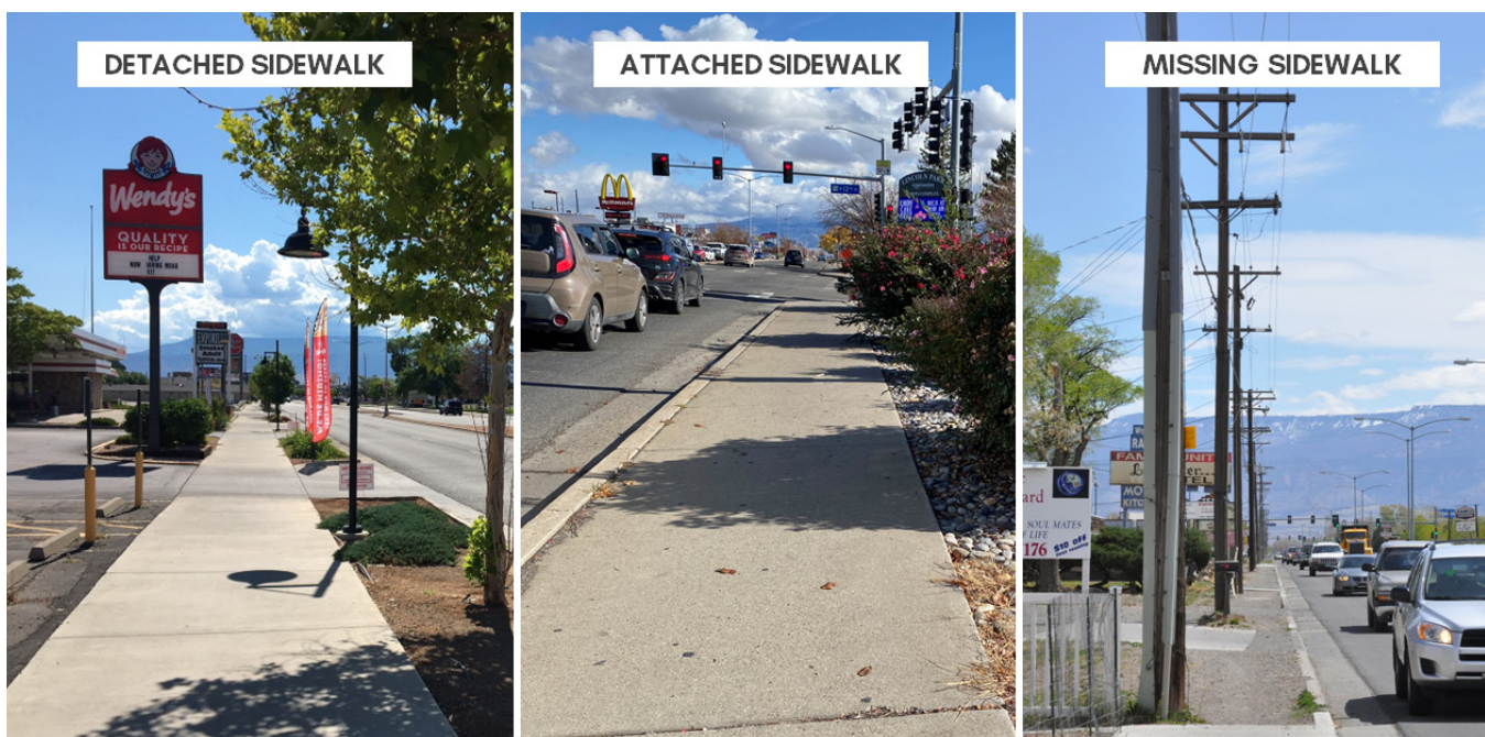
FIGURE 1: EXISTING SIDEWALK TYPES MAPPED IN GRAND JUNCTION
