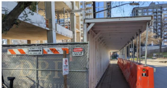
FIGURE 43: EXAMPLE OF COVERED WALKWAY AT CONSTRUCTION SITE
