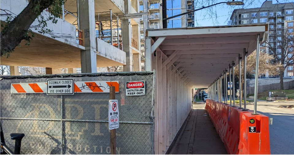
FIGURE 43: EXAMPLE OF COVERED WALKWAY AT CONSTRUCTION SITE
