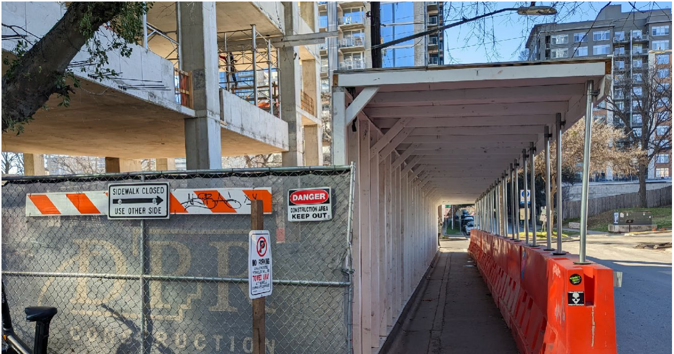
FIGURE 43: EXAMPLE OF COVERED WALKWAY AT CONSTRUCTION SITE
