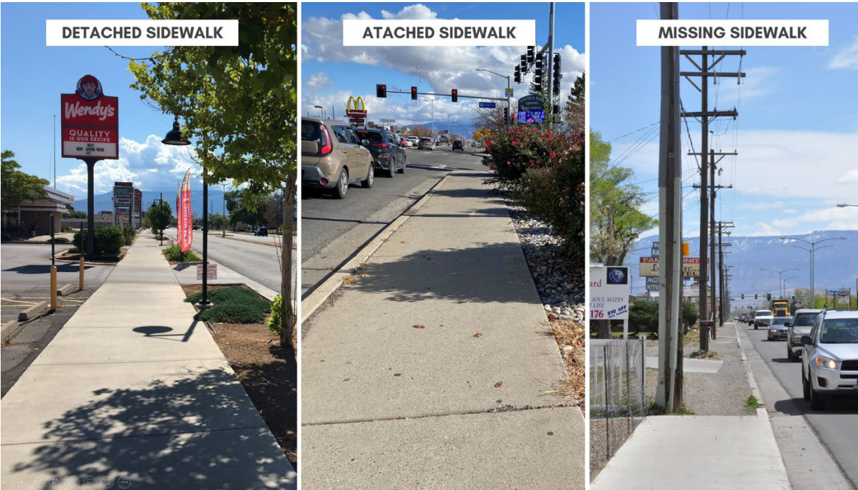
FIGURE 2: SIDEWALK CONDITION EXAMPLES
