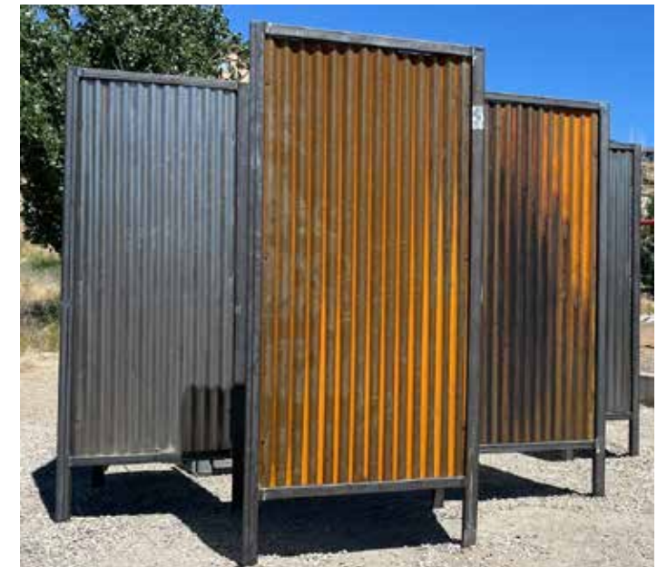
PORTO SCREEN STRUCTURE CITY OF GRAND JUNCTION
