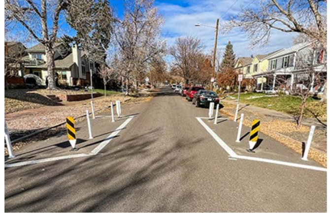
Retrofit Choker (source: City of Denver, Colorado)
