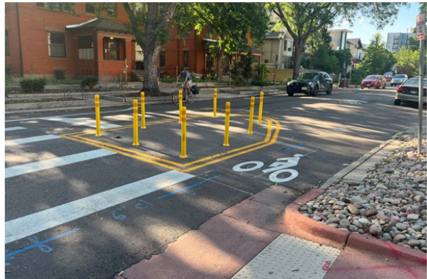
Retrofit Partial Closure
