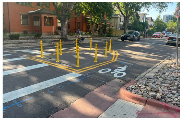
Retrofit Partial Closure
