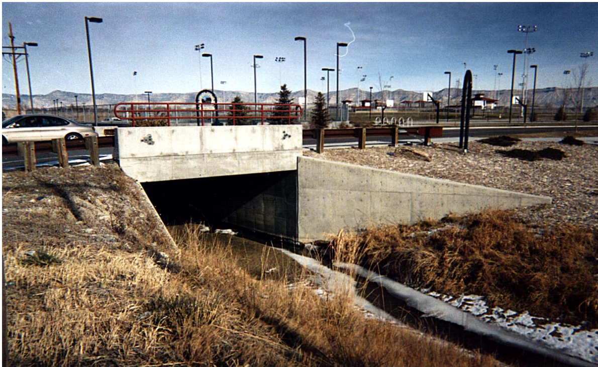
Leach Creek drainage structure near Canyon View Park
