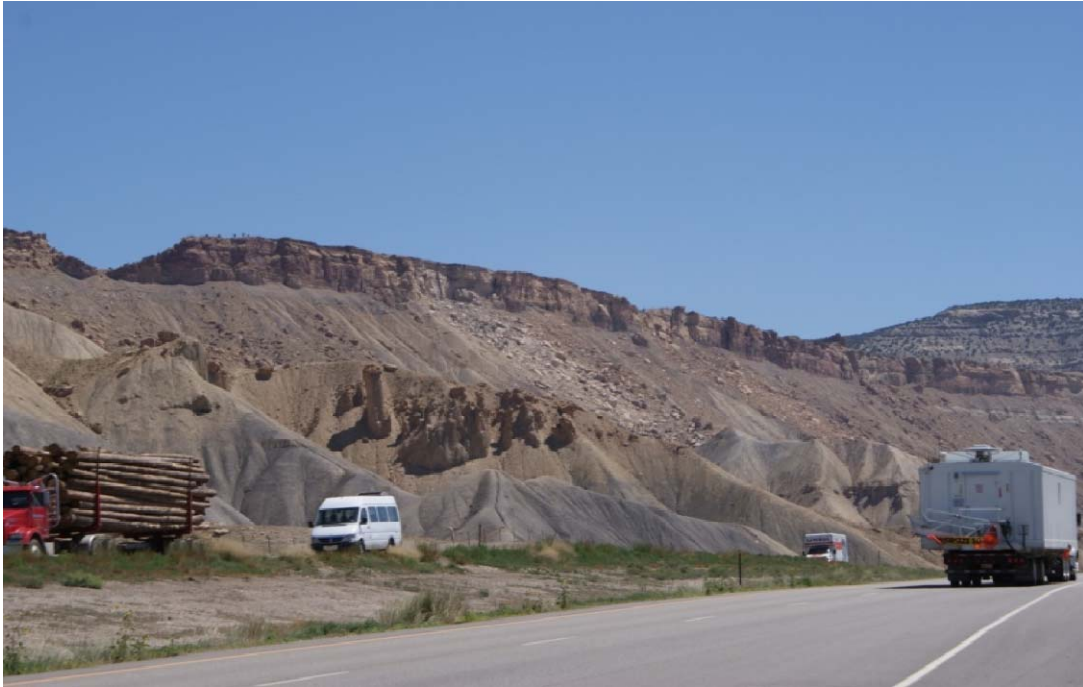
Figure 13: Rockfall West of Palisade Along Interstate 70
