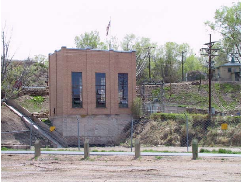
Redlands Power Canal and Power Station
