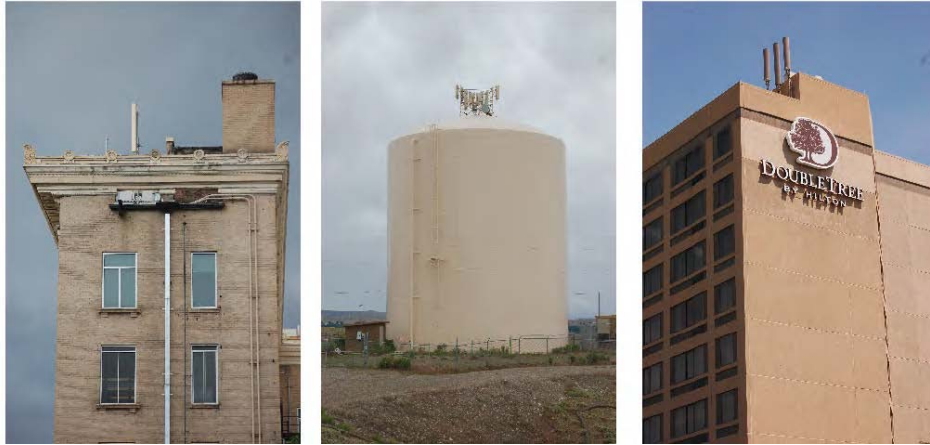
Figure 5: Examples of Nonconcealed Base Stations
