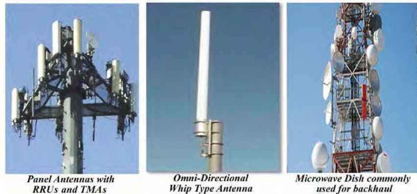
Figure 3: Examples of Panel, Directional and Microwave Antennas
