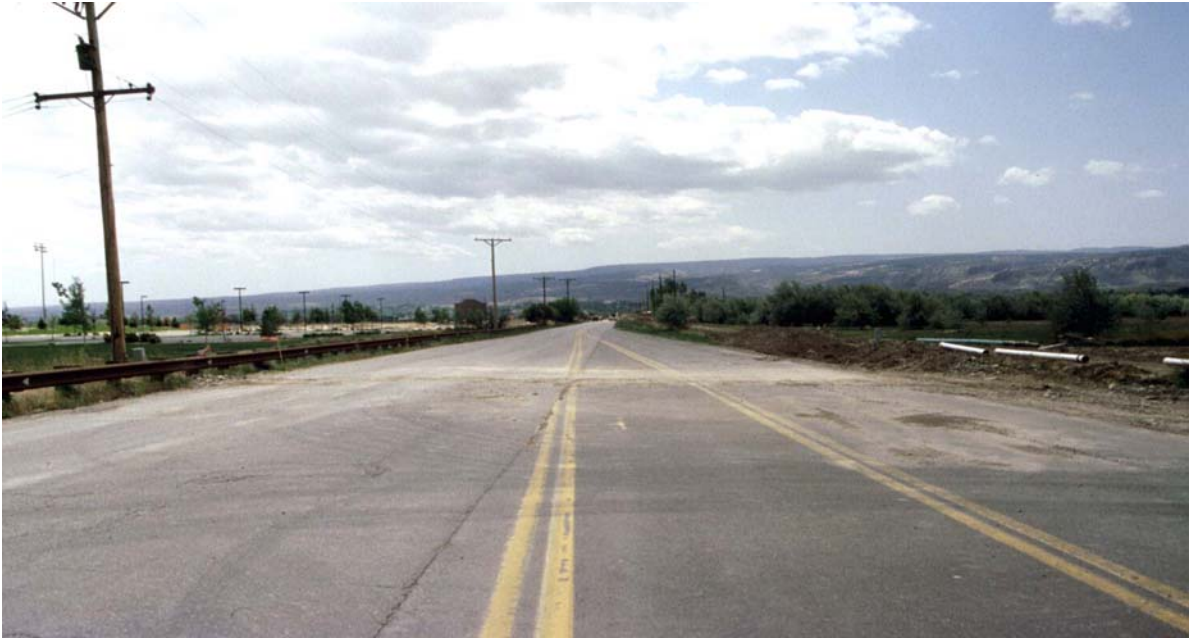
View to the Colorado Monument from 24 Road
