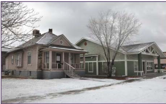
New Infill Development Building on Right
