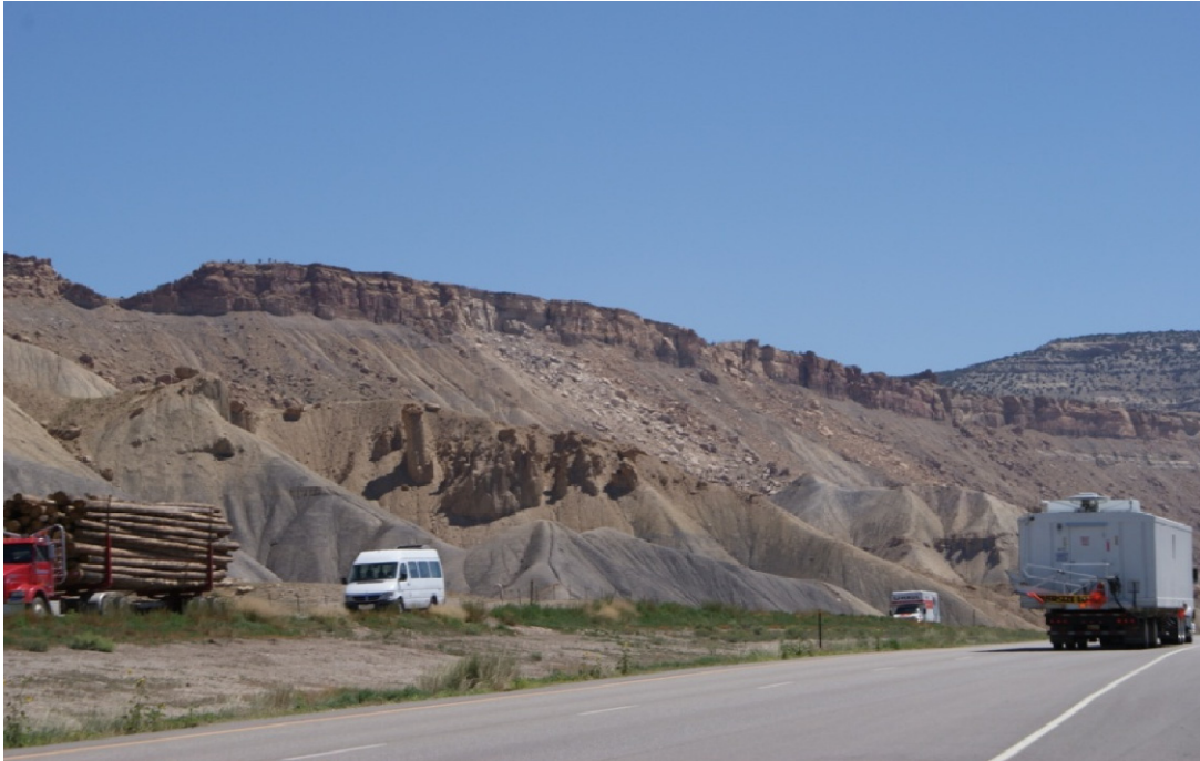
Figure 13: Rockfall West of Palisade Along Interstate 70
