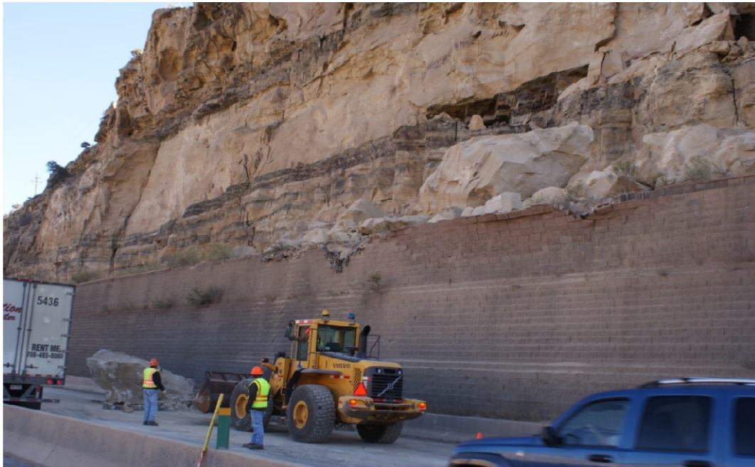
Figure 14: Rockfall Event in DeBeque Canyon at Beaver Tail Tunnel on Interstate 70
