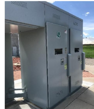
Primary switchgear.
