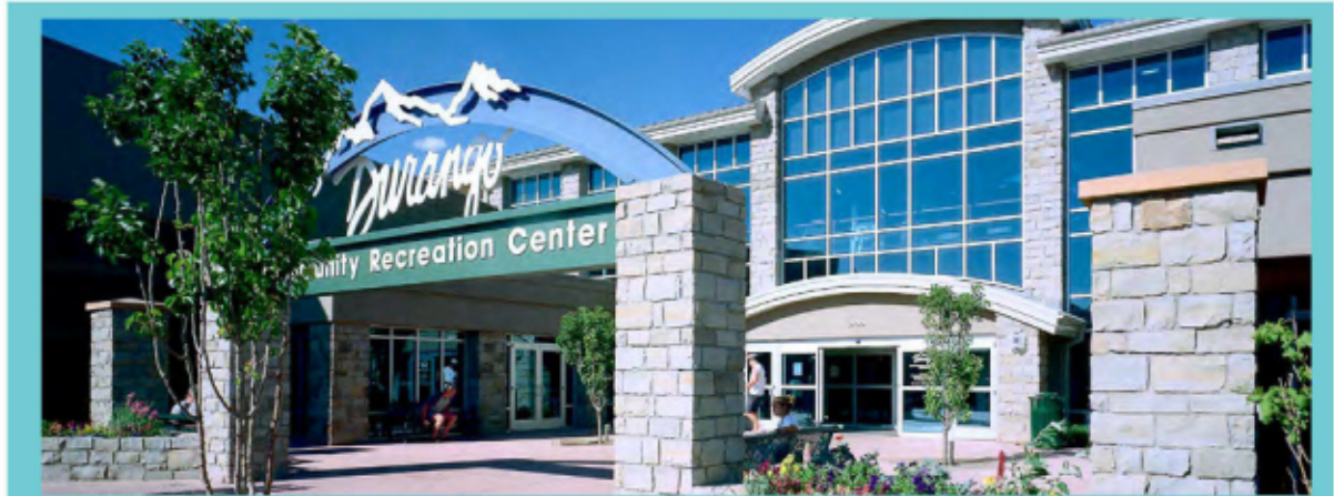
FCI and Barker Rinker Seacat have been completing recreation centers together for 23 years. Pictured above is our first recreation center we completed - The Duragno Community Recreation Center completed in 2002.
