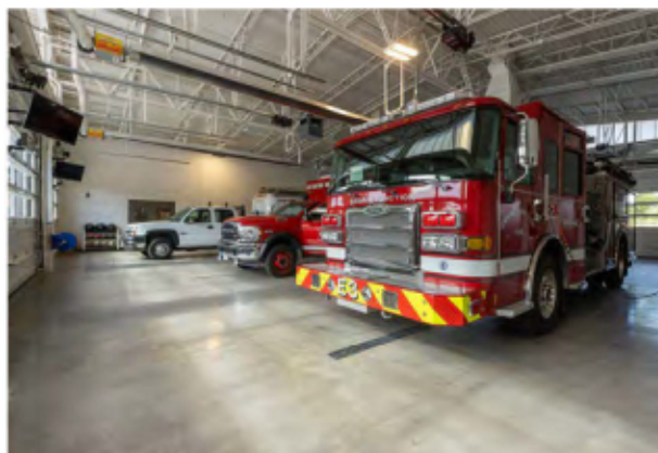
Fire Station No. 8, Grand Junction, CO
