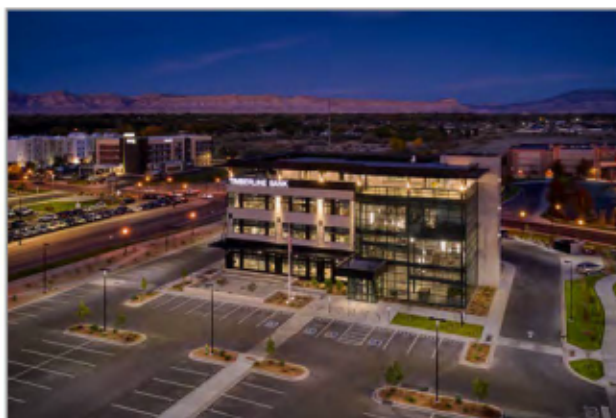
Timberline Bank, Grand Junction, CO
