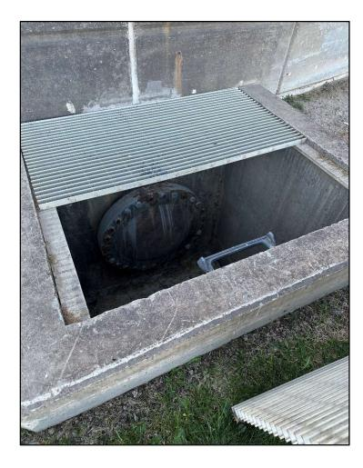
Picture shows Primary Anaerobic Digester 30" Manway cover. Secondary Anaerobic Digester Manway is nearly identical.
