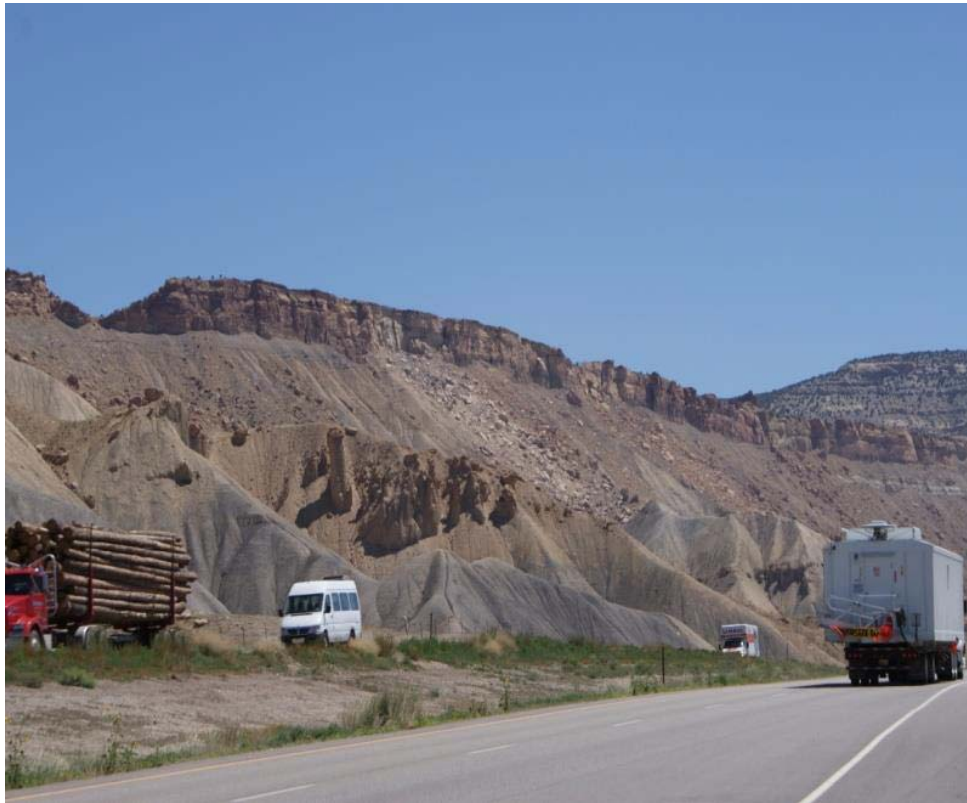
Figure 13: Rockfall West of Palisade Along Interstate 70
