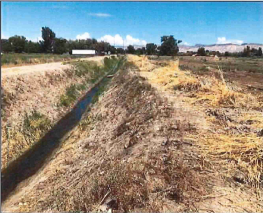
Photo 4. No name drain, view north along west boundary (August 2022)
