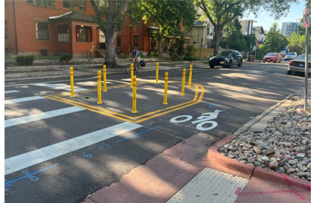
Retrofit Partial Closure
