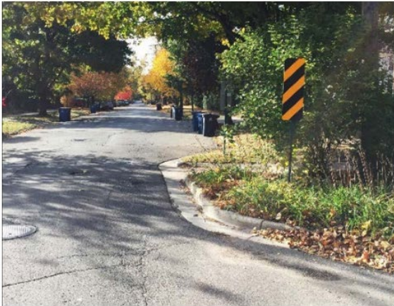
Permanent Choker (source: City of Ann Arbor, Michigan)
