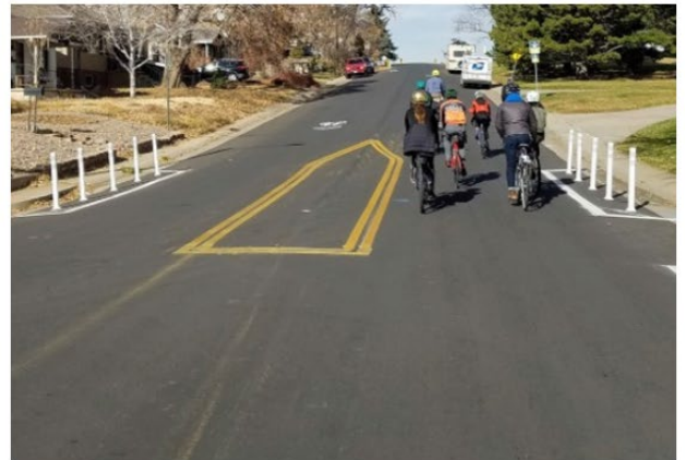
Retrofit Median (source: City of Denver, Colorado)
