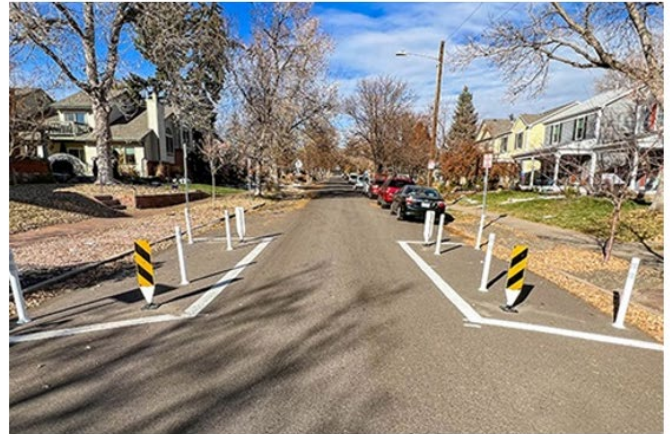
Retrofit Choker (source: City of Denver, Colorado)
