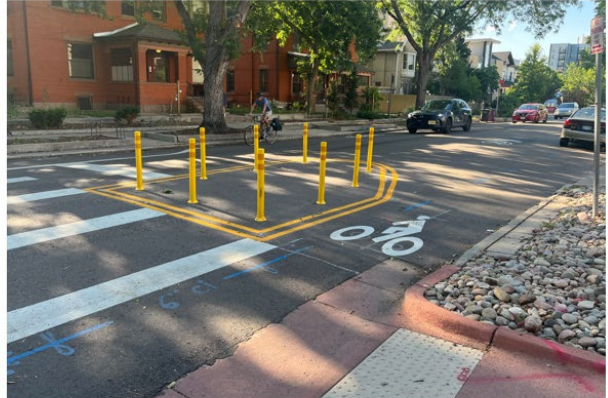
Retrofit Partial Closure
