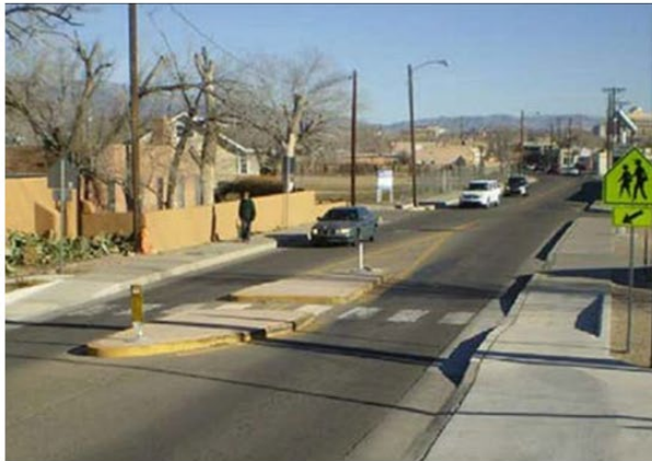
Permanent Median (source: James Barrera, Harrocks New Mexico)
