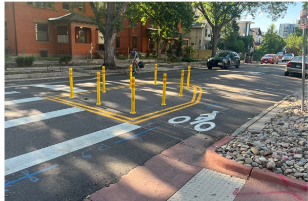
Retrofit Partial Closure
