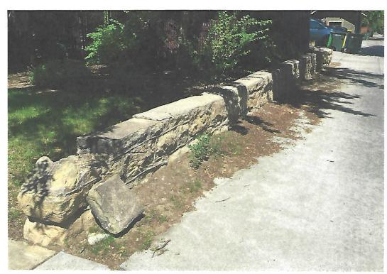
CONDITION OF 20" TALL STONE AND CONCRETE WALL, CRUMBLING,
