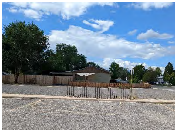
Picture 3, Bike rack blocking sidewalk
