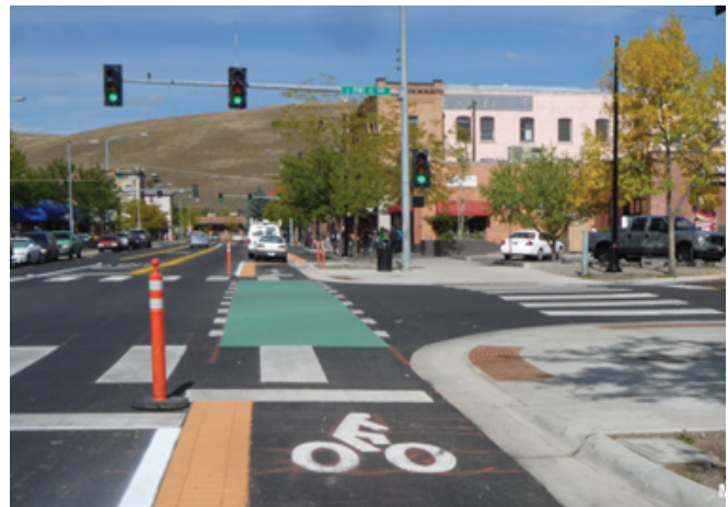
FIGURE 28: RECESSED STOP BAR
