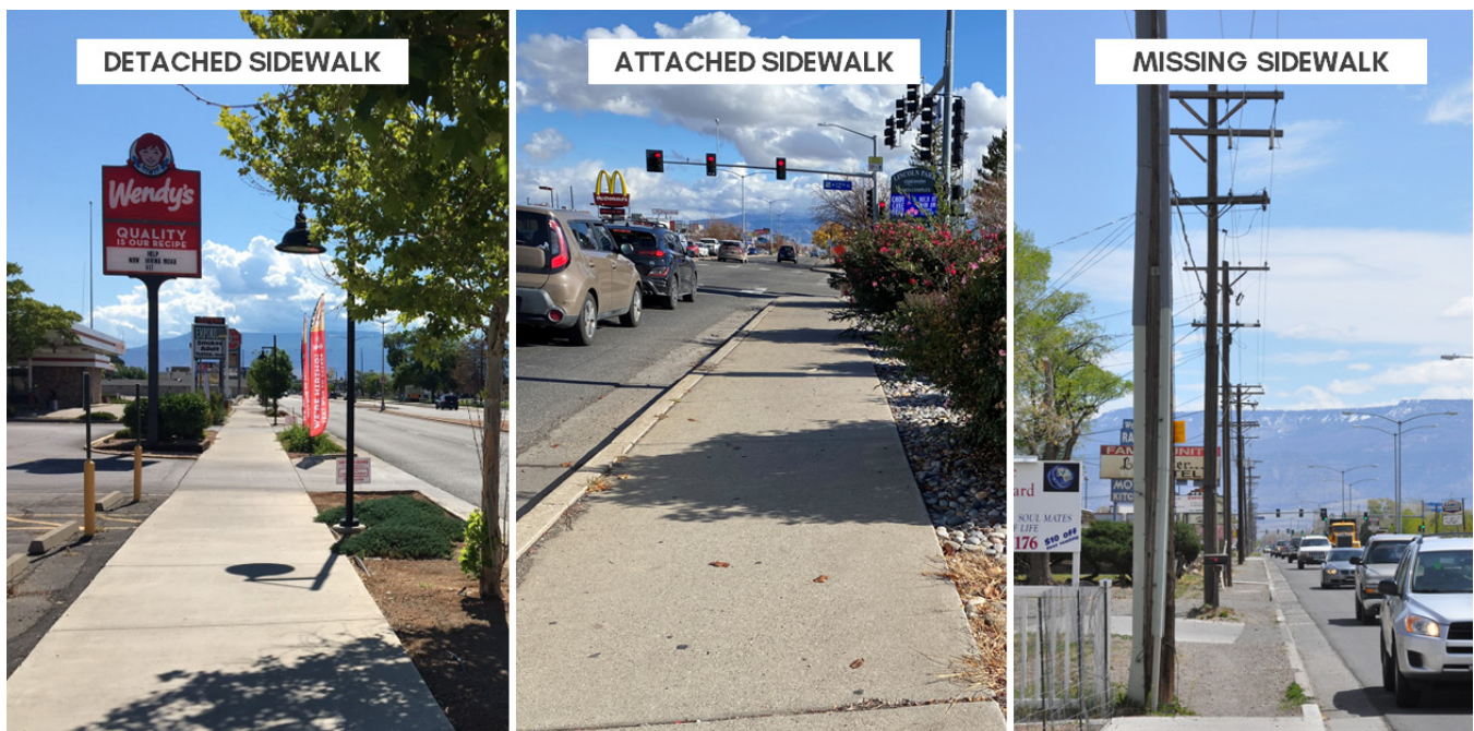
FIGURE 1: EXISTING SIDEWALK TYPES MAPPED IN GRAND JUNCTION
