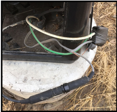
Sample UG fuse/fuse holder
