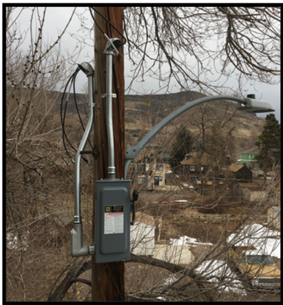
Sample OH switch/disconnect system:
