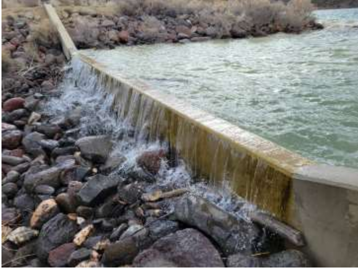
Spillway activation photo taken 6Mar2023.
