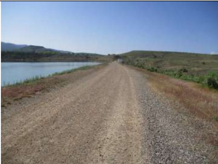
View of the crest from the right side.
