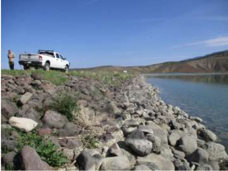
Looking across the upstream slope toward the right abutment.
