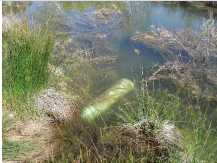
Submerged toe drain.
