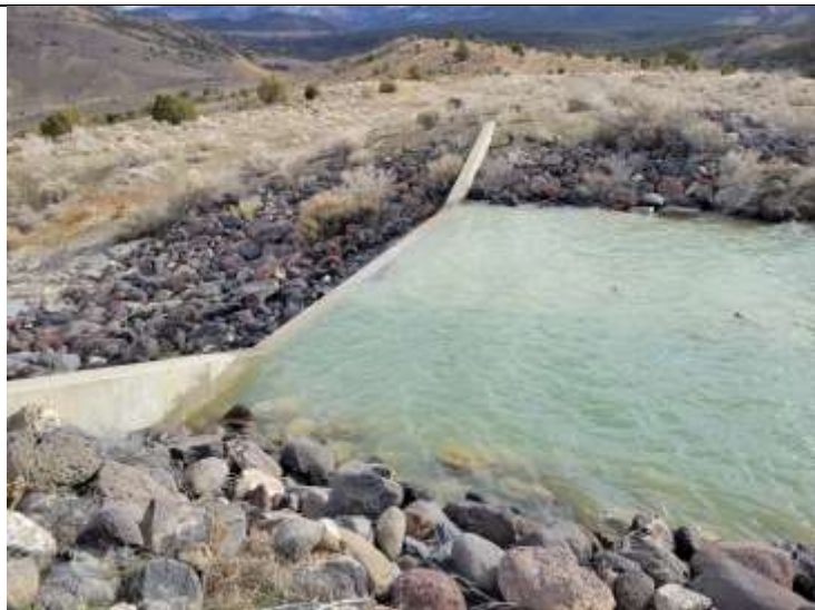
Spillway activation photo taken 6Mar2023.
