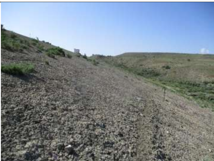
Looking across the downstream slope from the right side.
