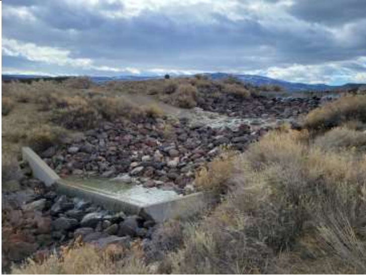
Spillway activation photo taken 6Mar2023.
