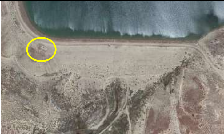
Google imagery showing downstream slope. Seepage area identified.
