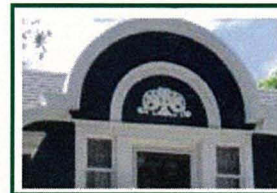
Example of a Parapet
